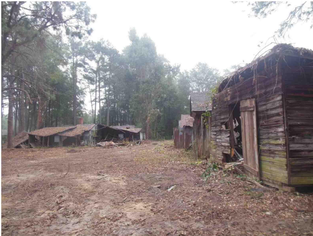
Site view from West looking due east
