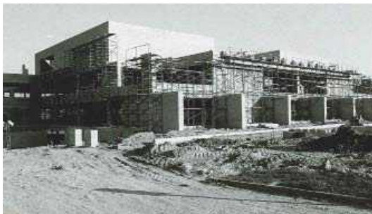
Concrete masonry unit solid walls
