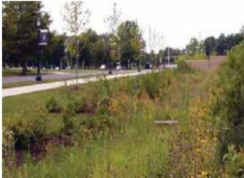
Bioswale along street
