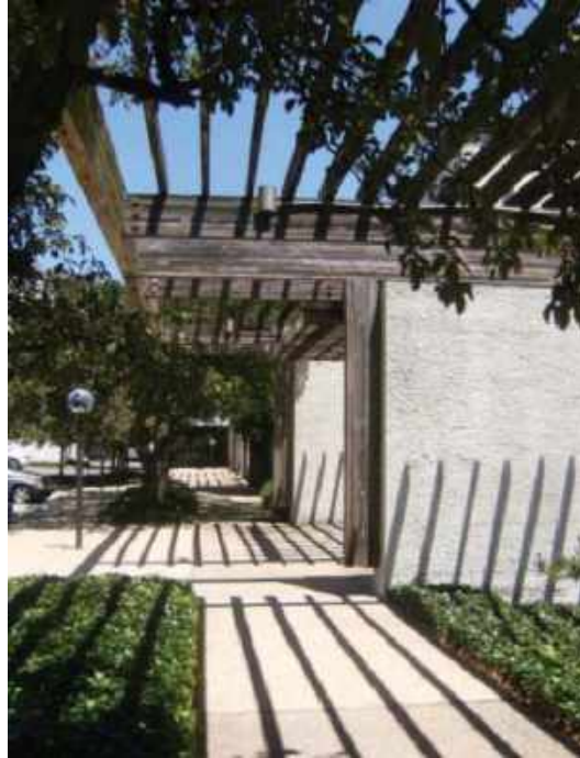
Wood Trellis at West Facade
