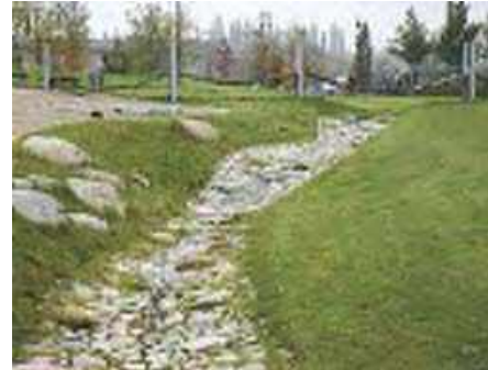
Example of surface Bioswale
