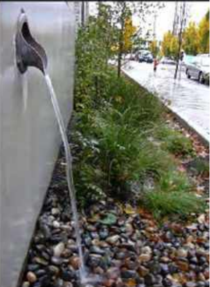
Rainwater is drained into bioswale
