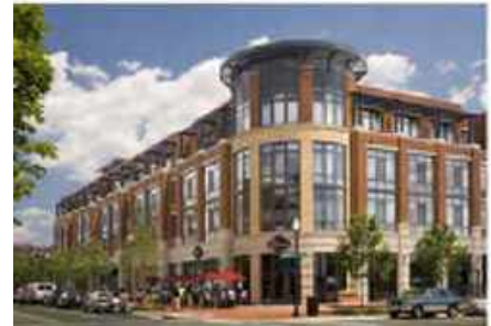
Example of columns overwhelming retail fronts (above)
