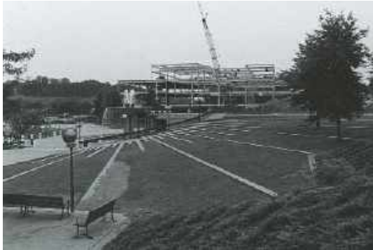
Steel framed building structure, under construction
