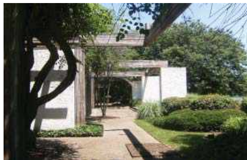
East Facade, with Lake Level Terrace
