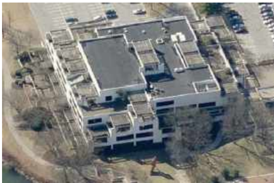
Overhead view from North-East
