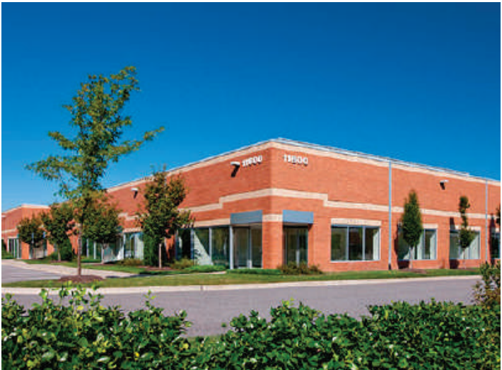
Baltimore Crossroads existing office space
