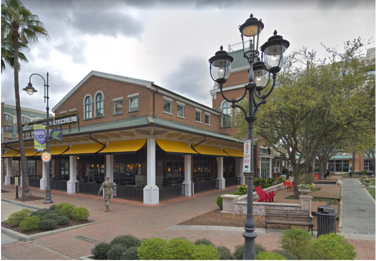
Precedent - Commercial Building - Baton Rouge, LA Credit: Google Maps Street View
