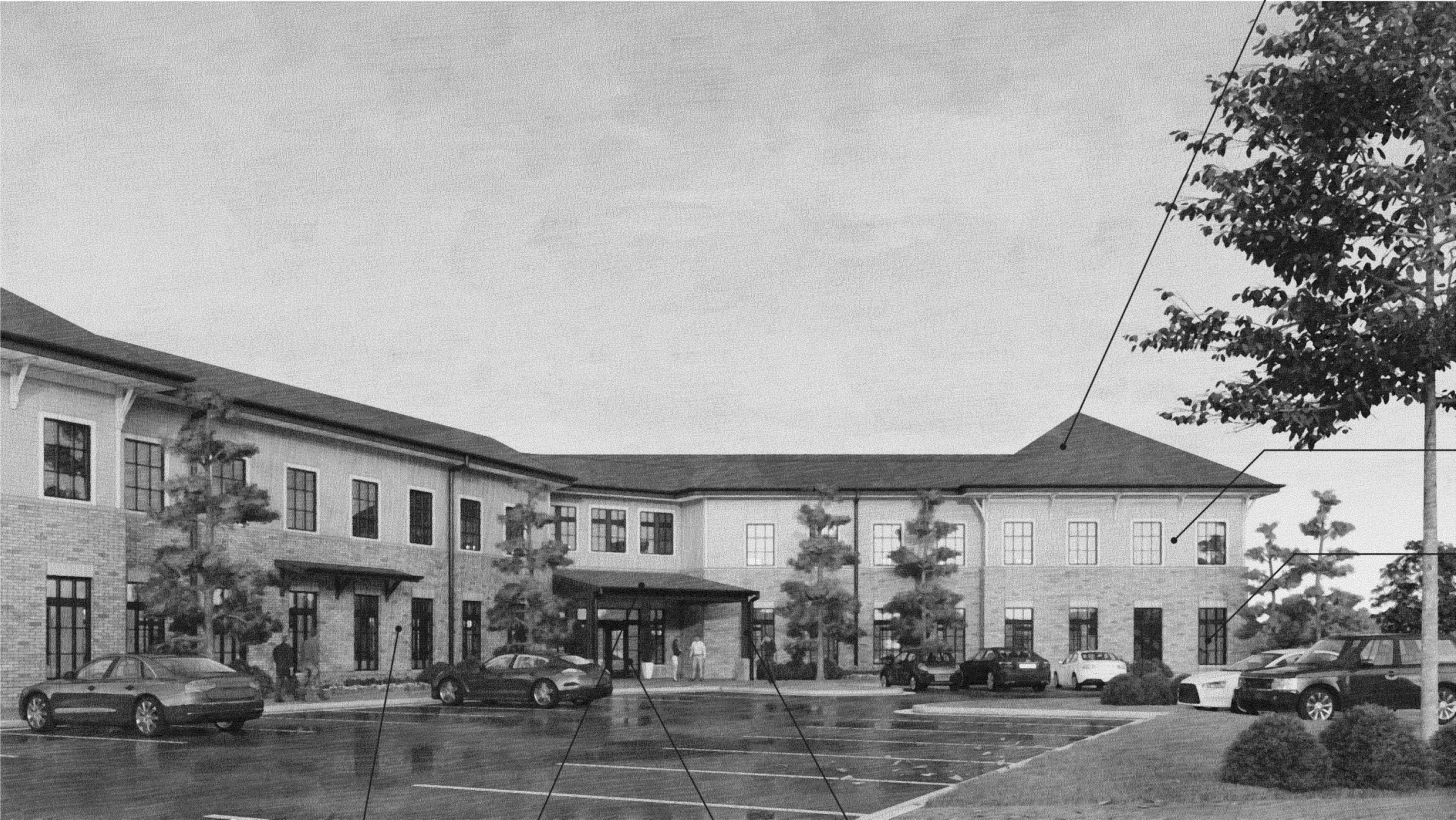
02 - VIEW TO ENTRANCE
