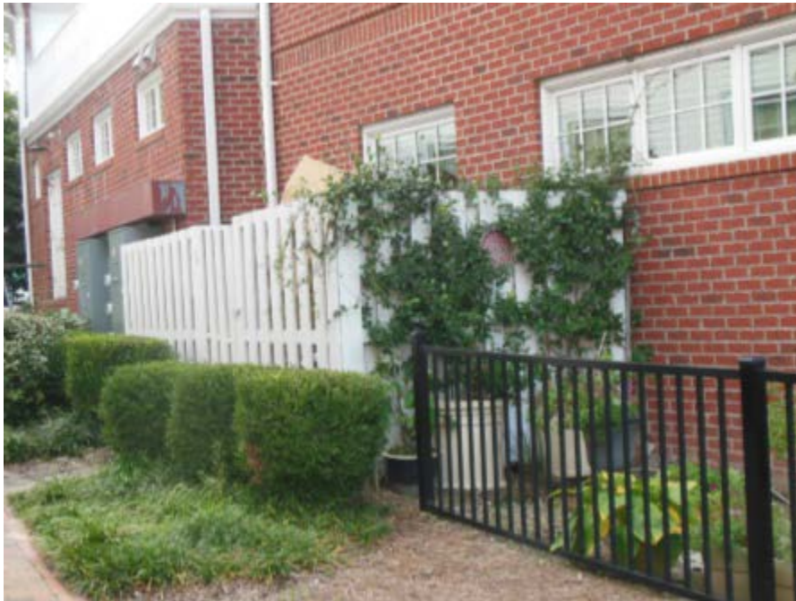
Screened commercial utility area
