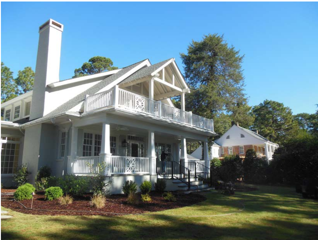
Rear porch and balcony addition
