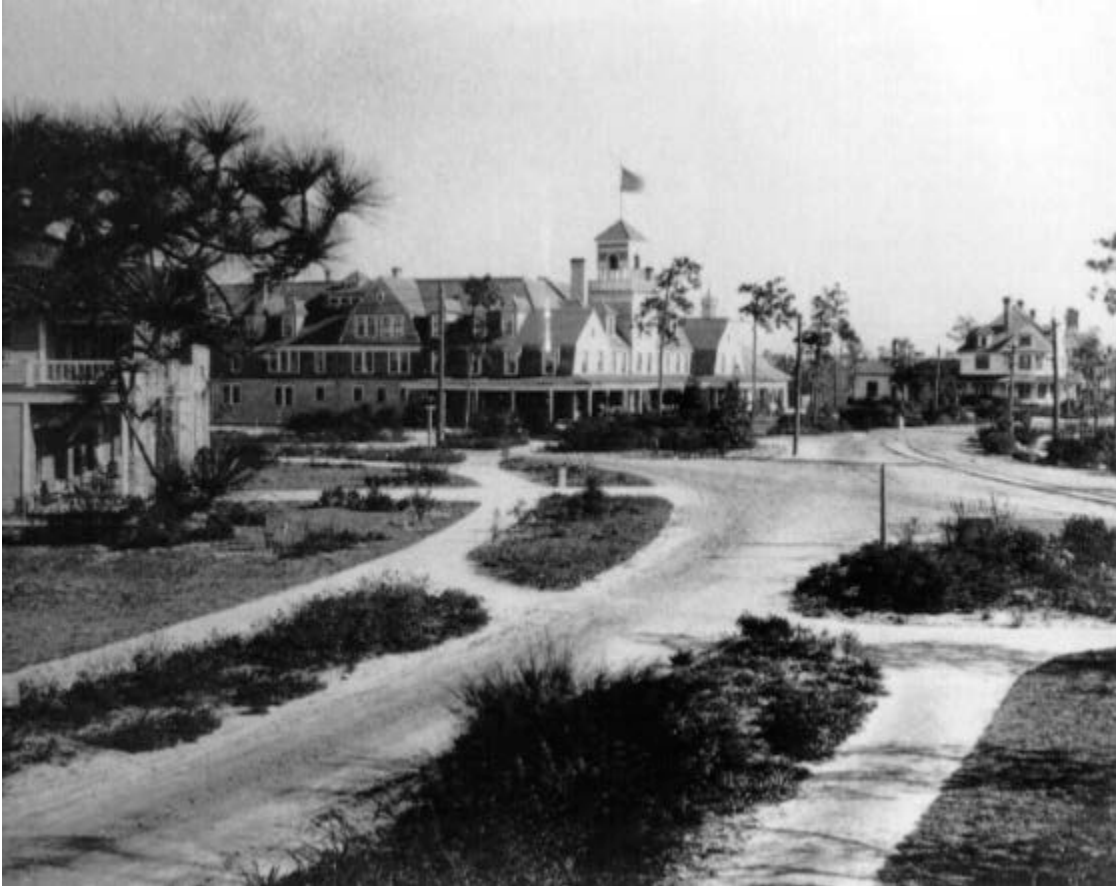
1920s Photo of clay paths and street-scaping
