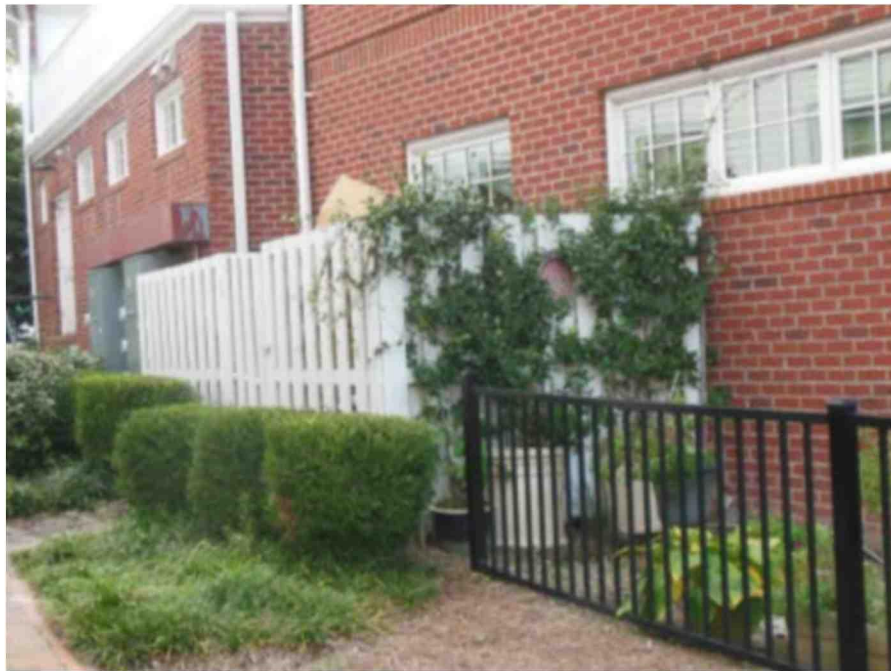
Screened commercial utility area
