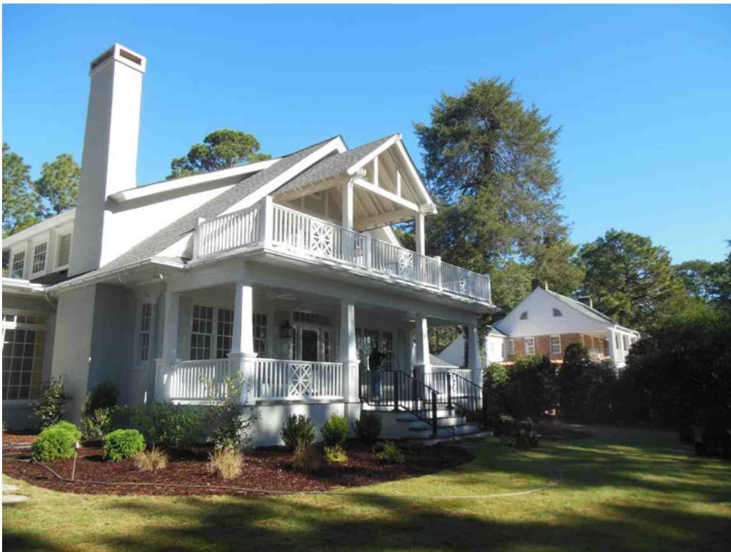
Rear porch and balcony addition
