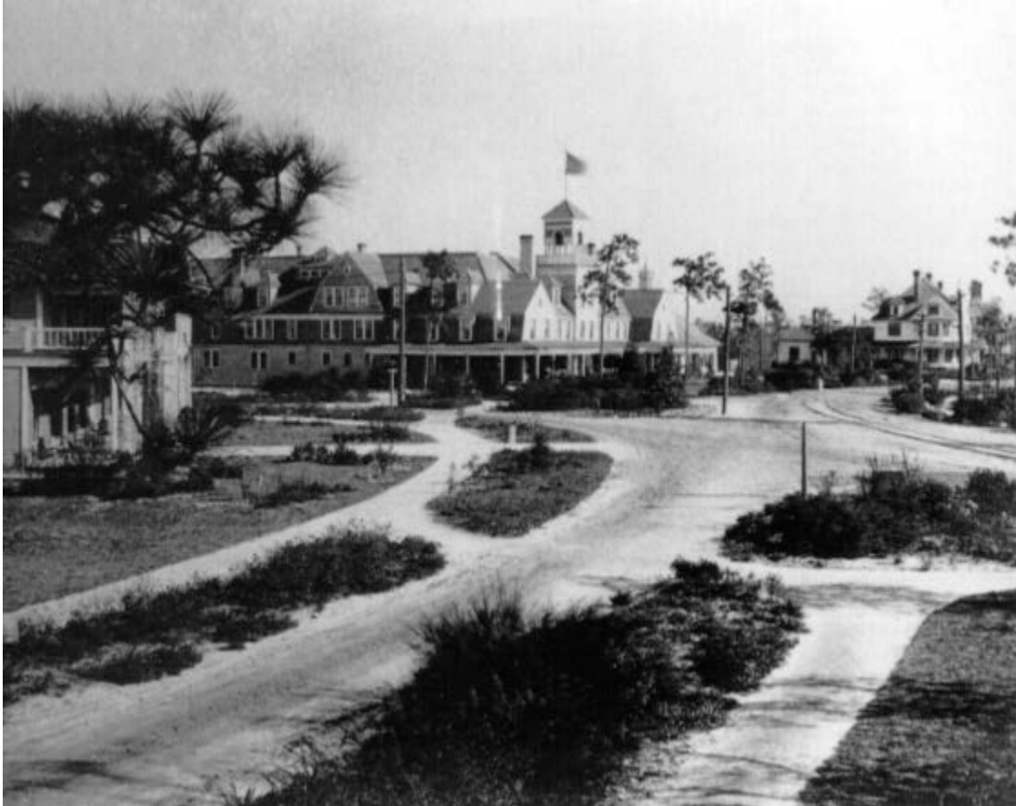
1920s Photo of clay paths and street-scaping
