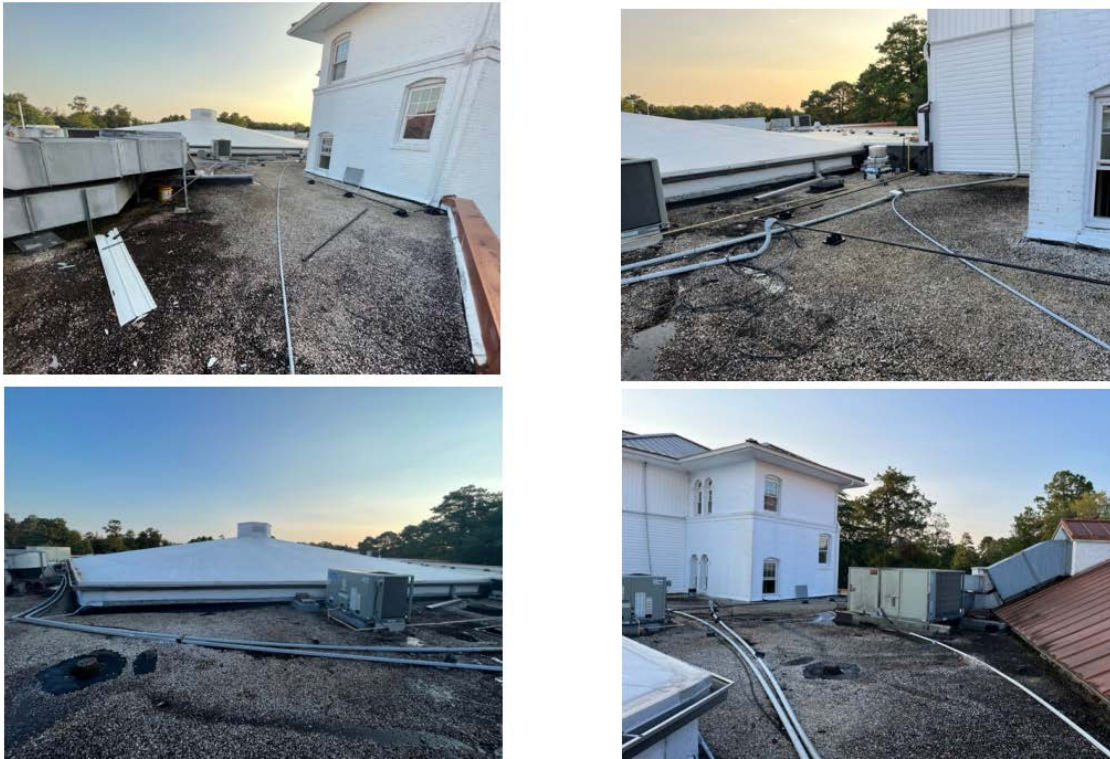
Pictures of the gravel tar roof at the Cardinal Ballroom:
