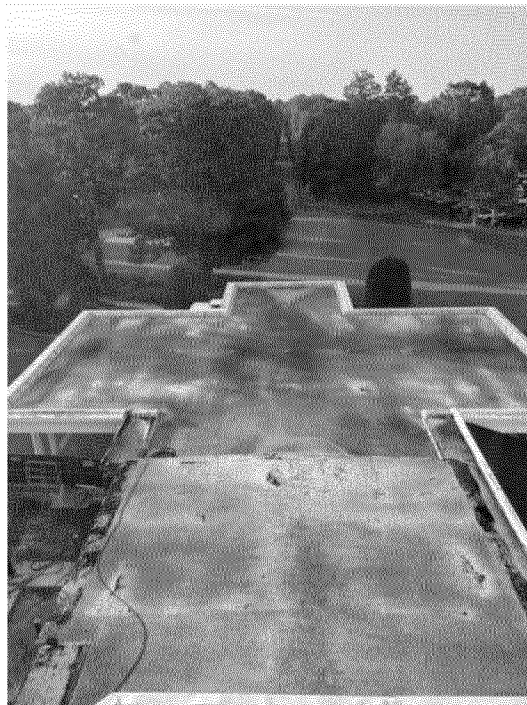
The flat rubber roof at the Carolina main entry lobby and porte-cochere location:
