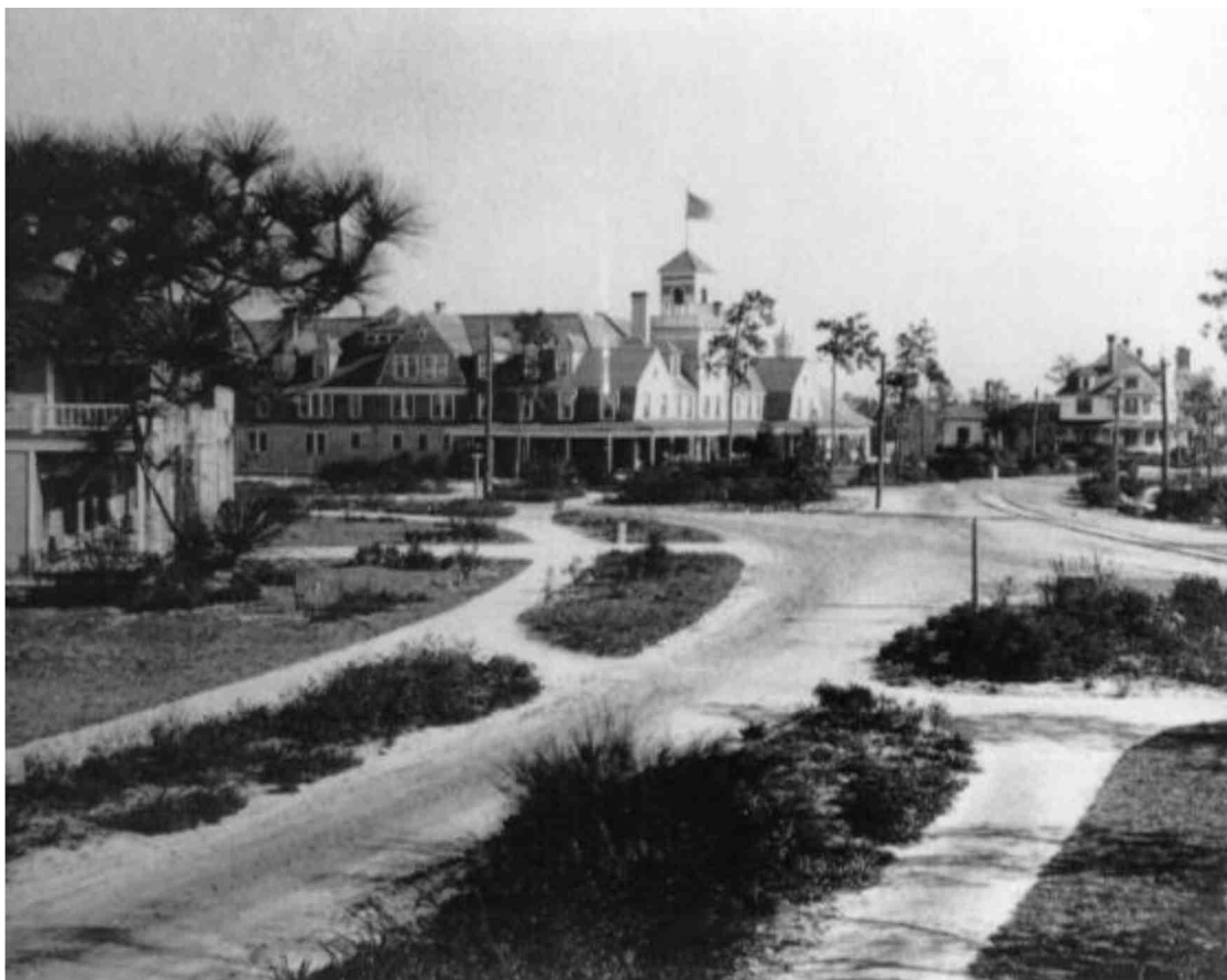
1920s Photo of clay paths and street-scaping
