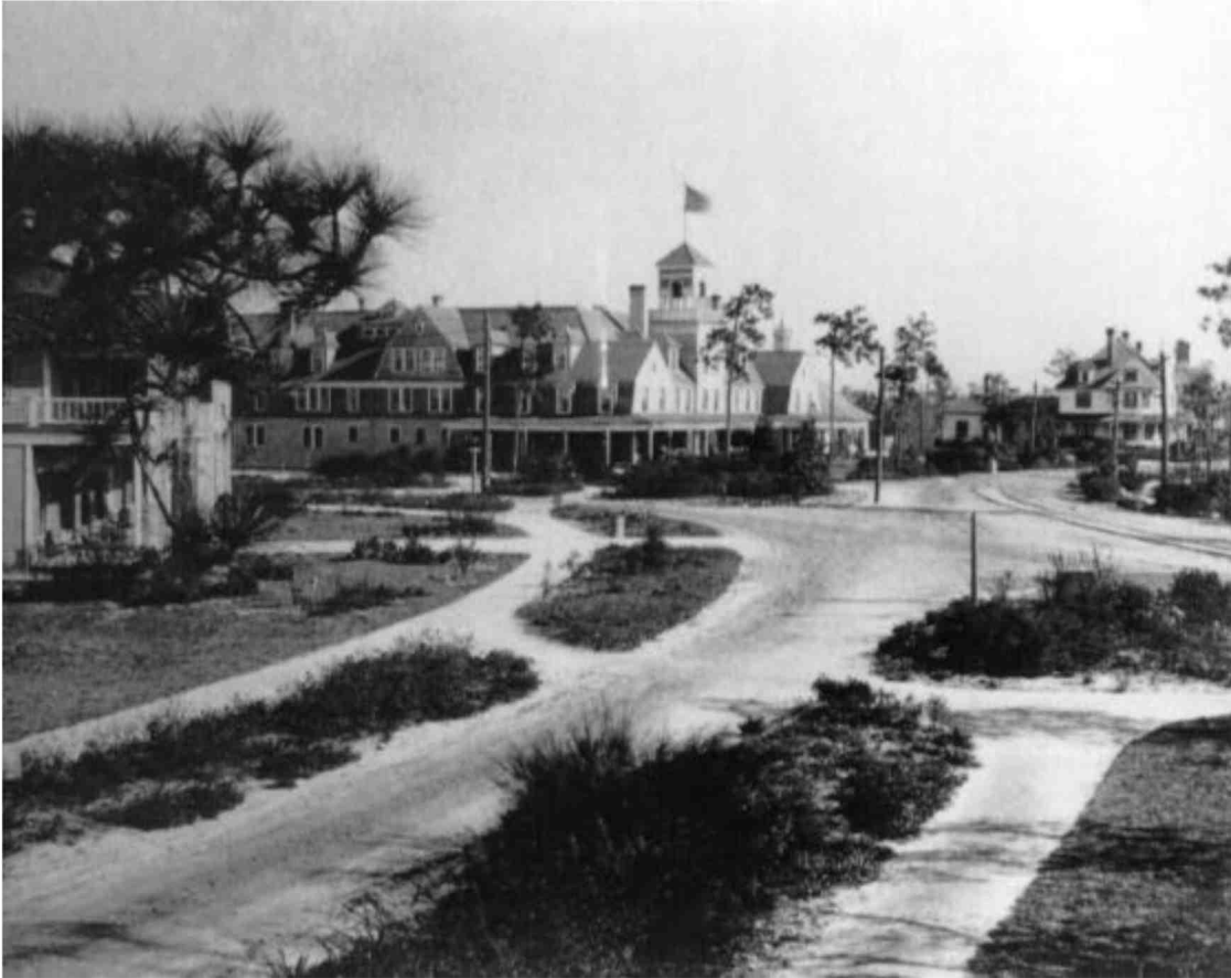
1920s Photo of clay paths and street-scaping
