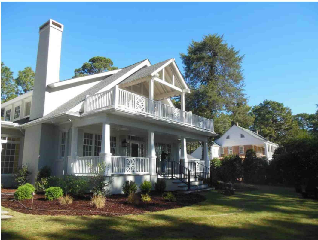
Rear porch and balcony addition
