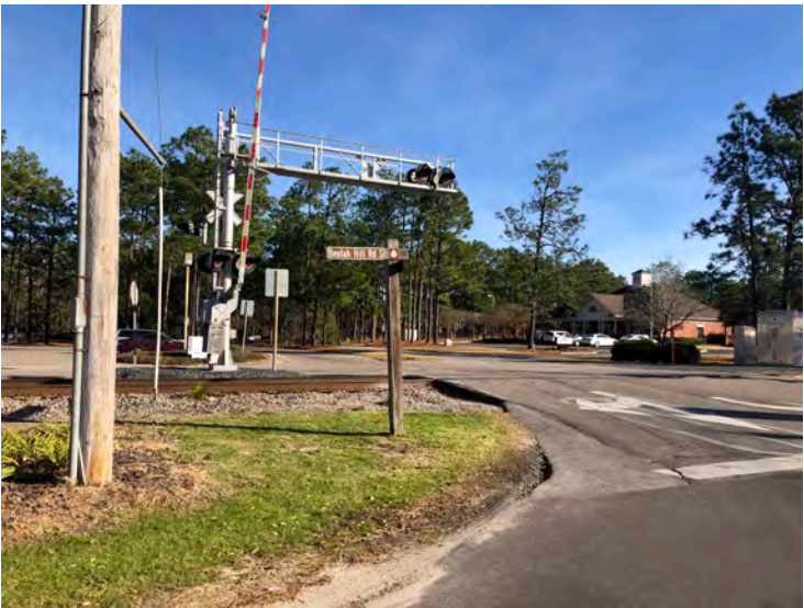
Blake Blvd Railroad Crossing Source: Design Collective
