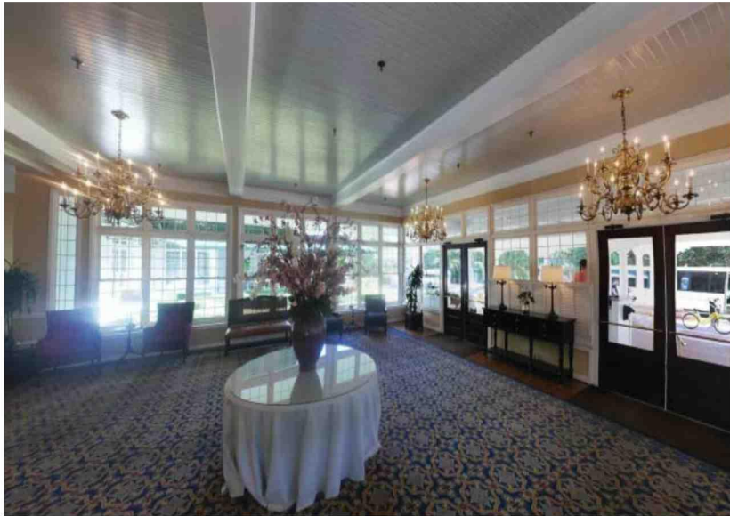
Existing Doors and Windows
