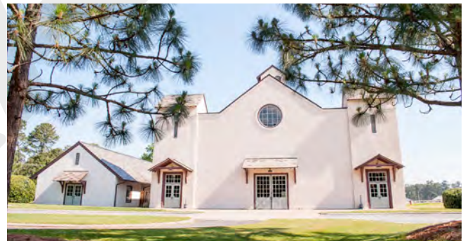
Fair Barn Facade/Village of Pinehurst
