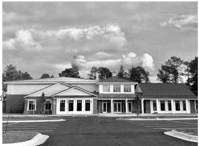
^ Canon Park Community Center/Village of Pinehurst
