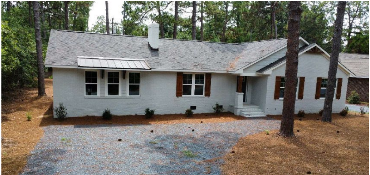
Photo of main residence with overhang and windows to have shutters added
