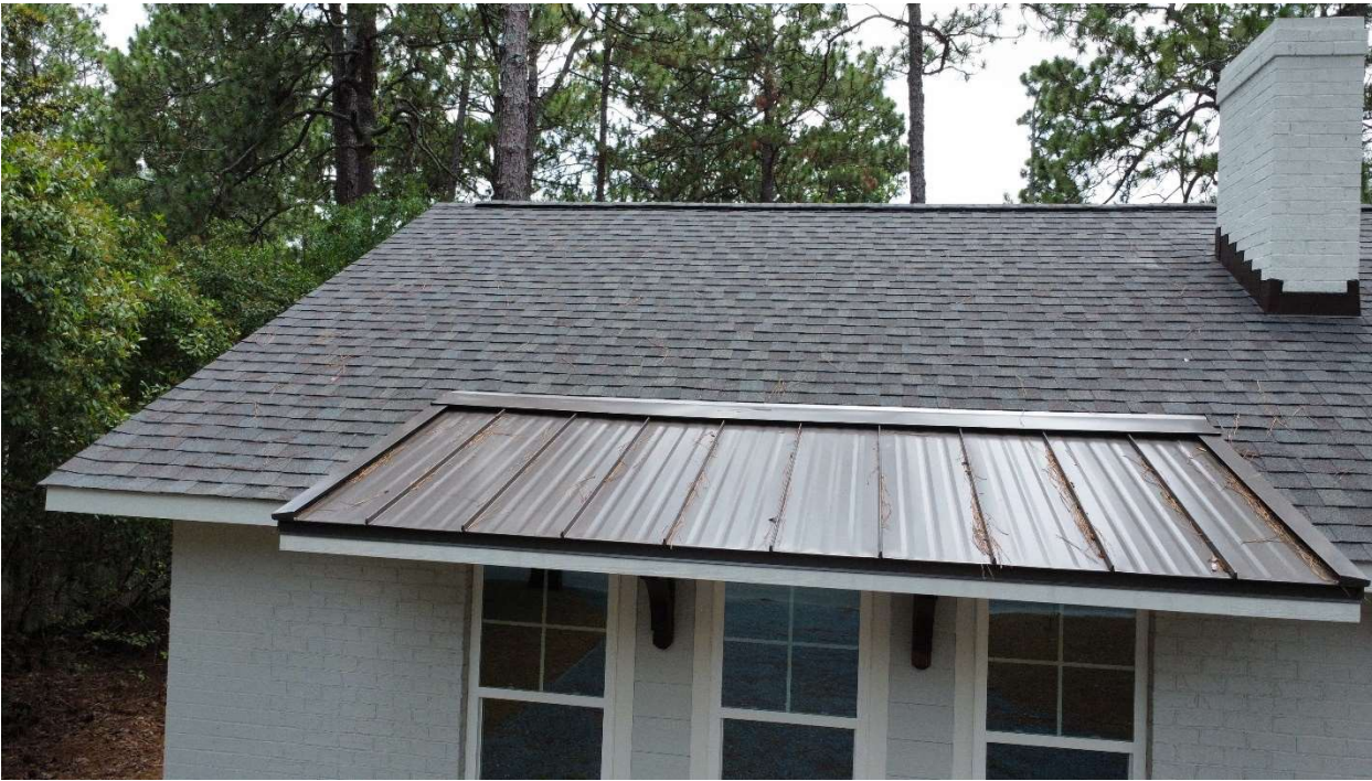
Photograph of new roof.
