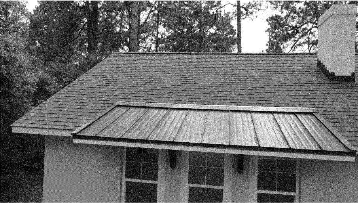
Photograph of new roof.
