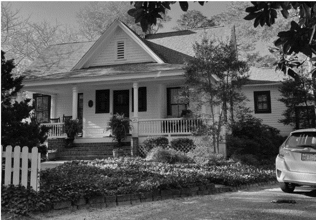
Photo of main residence
