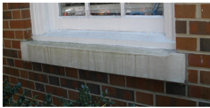
Precast Window Sills, 1961 & 1991
