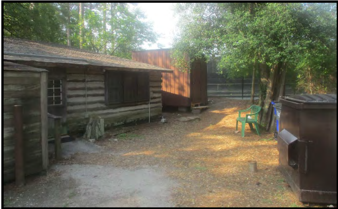
Photo #3 - This is the north wall at the rear.
