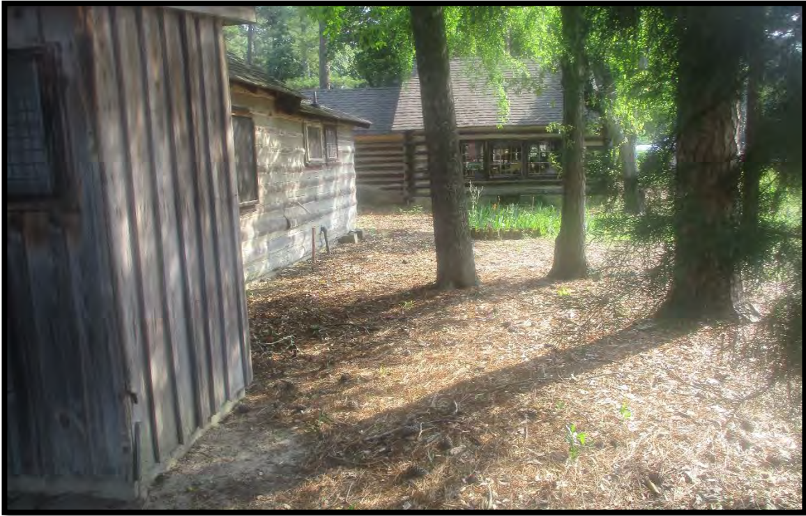
Photo #5 - This is the south face of the building that faces the two south drainage ponds.
