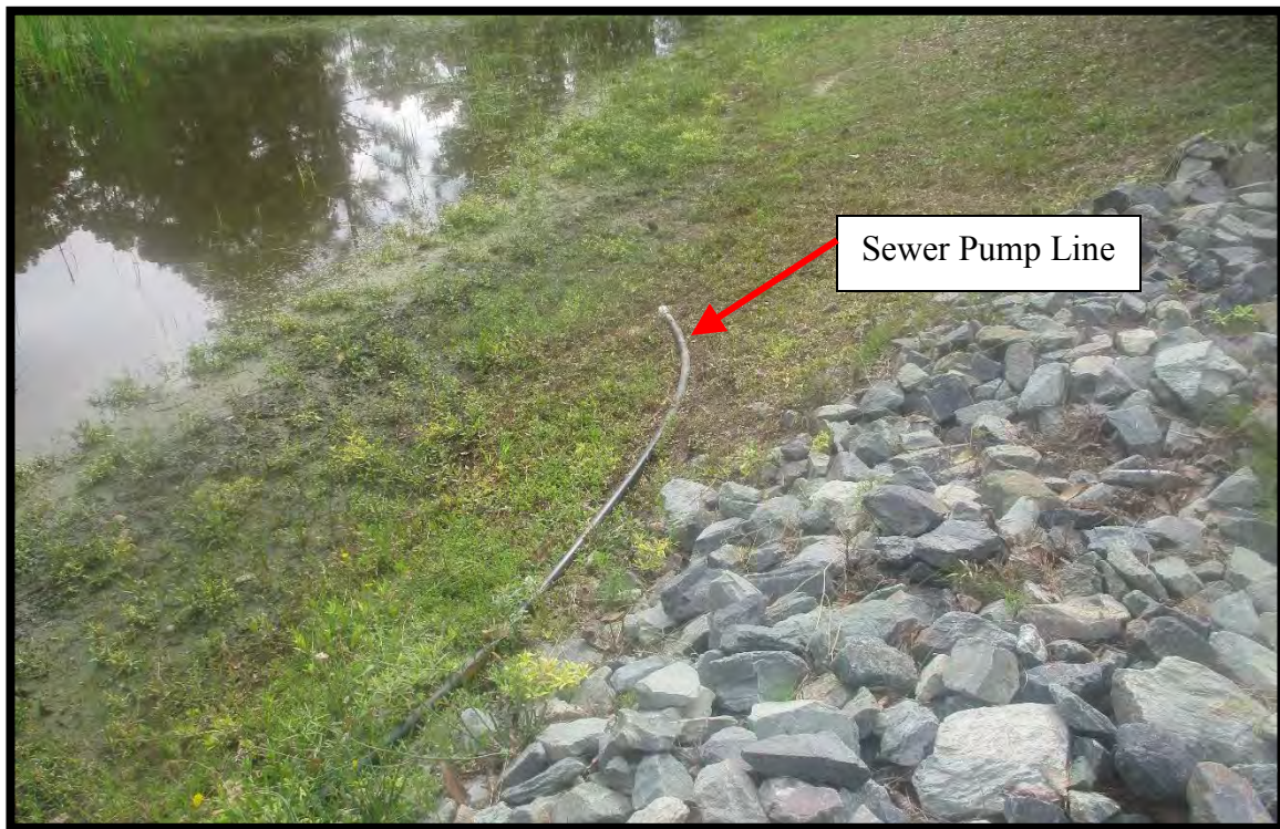
Photo #11 – There is a sewer pump line that appears to pop out of the ground at the upper pond and then goes back into the ground at the lower pond.
