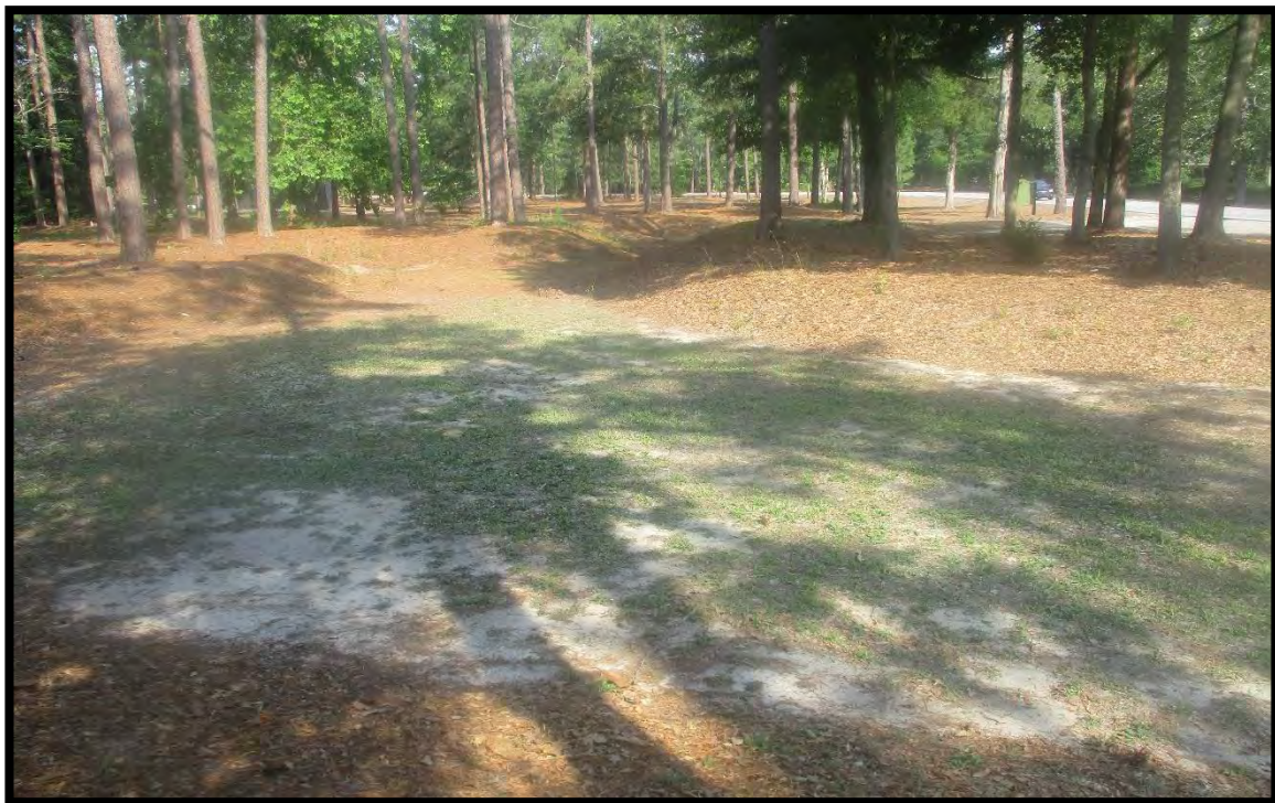
Photo #12 - This is the north side drainage pond. It collects water from the neighboring streets but has no outlet.
