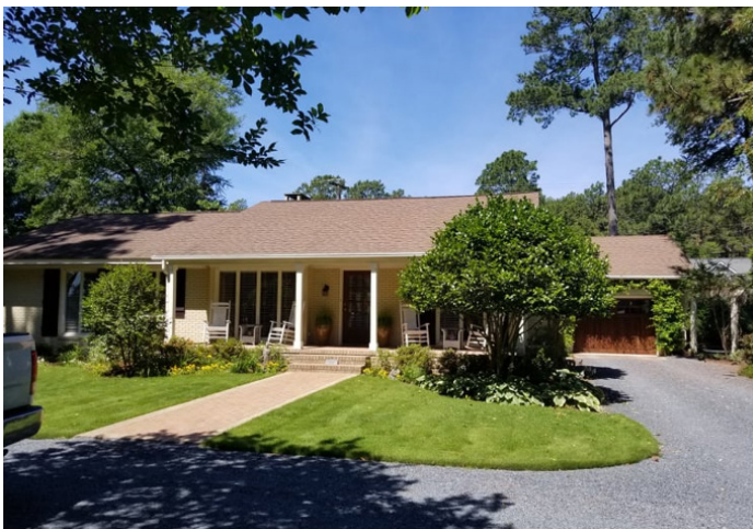
Existing Roof Color
