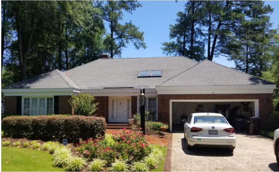
Existing similar color and material roof across subject property (40 Laurel Rd.)
