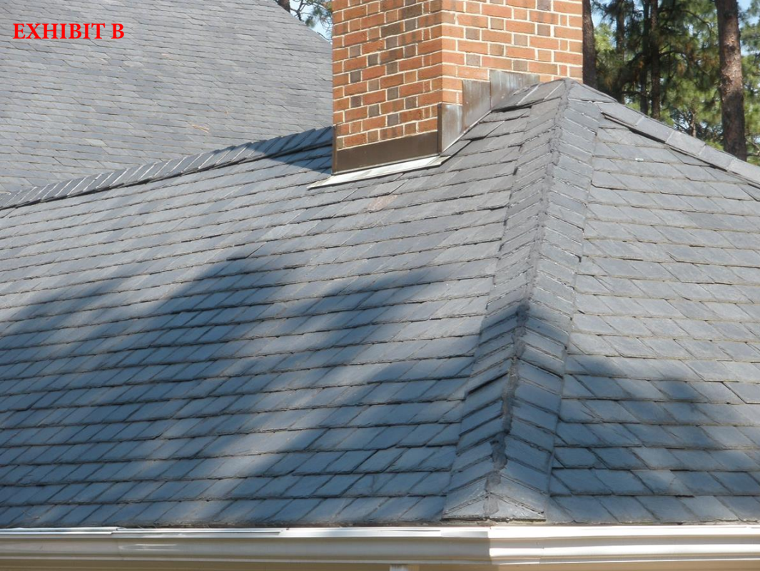
Slate Roof, 1961 shown in picture.
