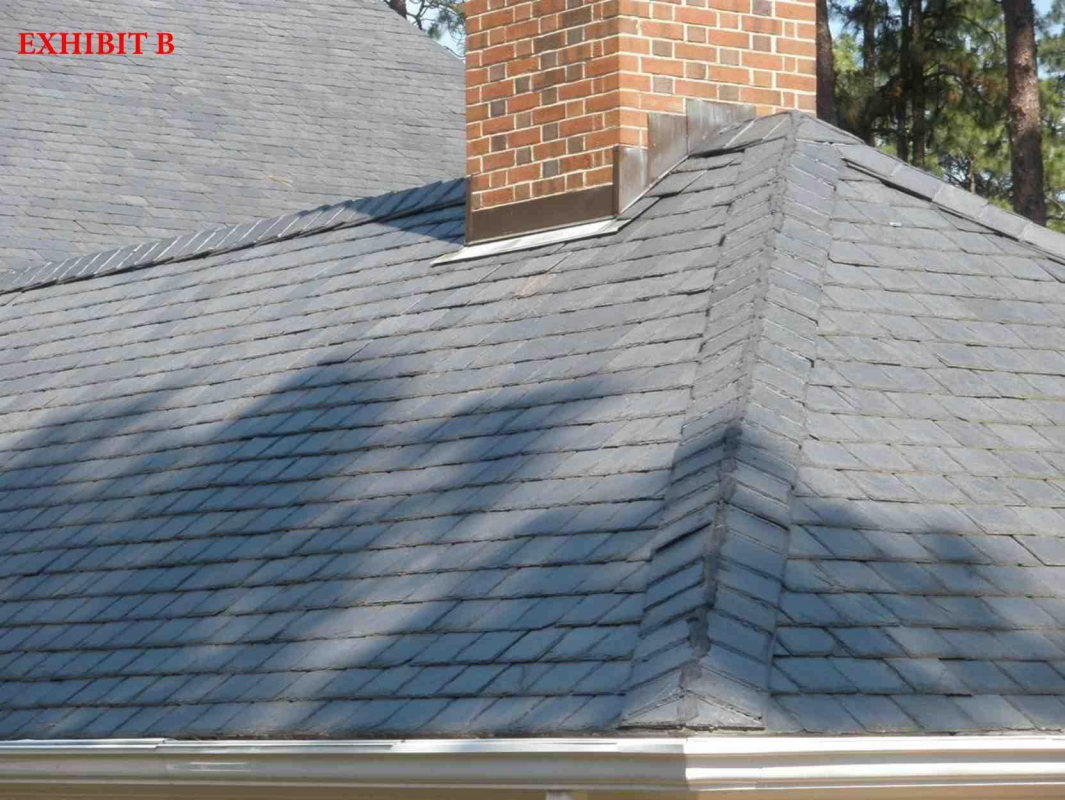
Slate Roof, 1961 shown in picture.
