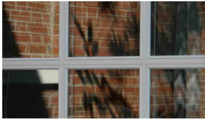
Clad Wood Window Grid, 1991
