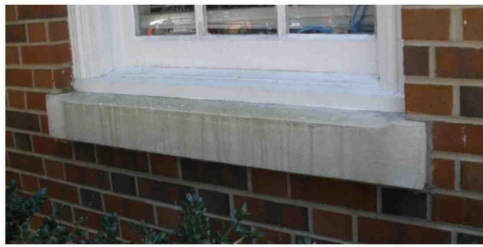
Precast Window Sills, 1961 & 1991
