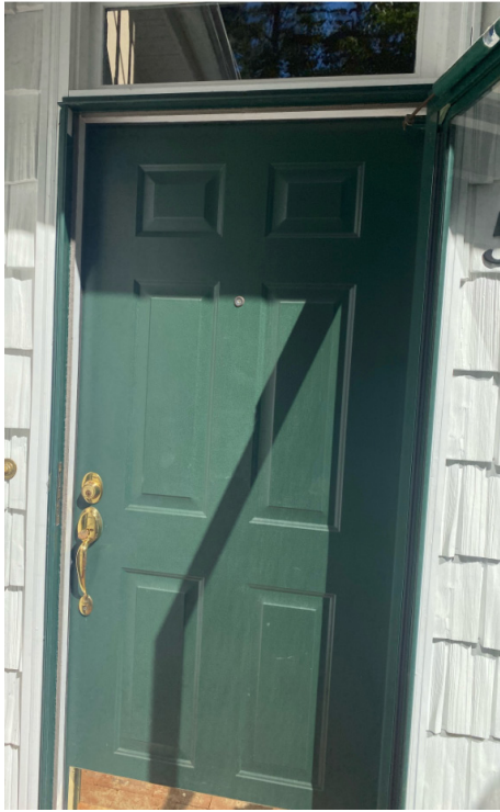
Existing Front Door
