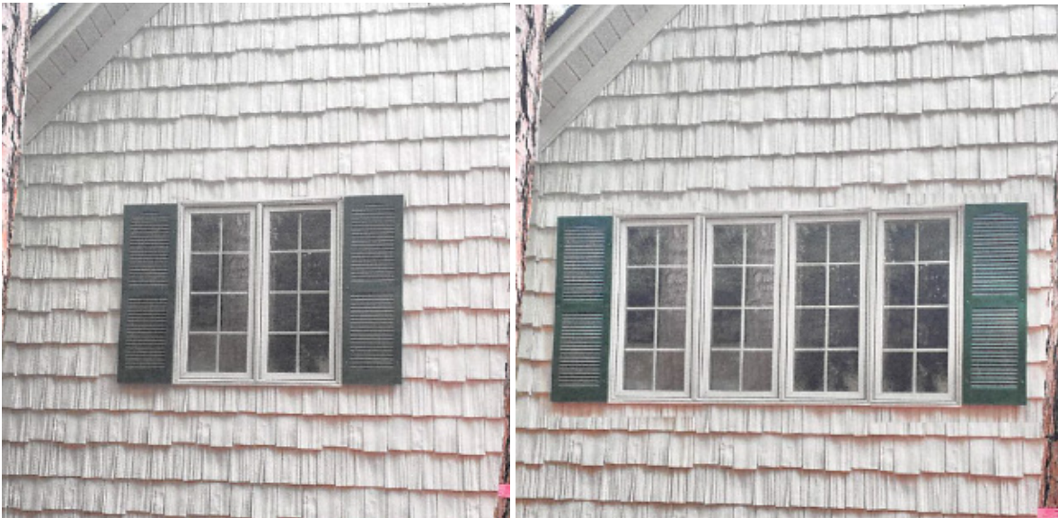
Existing Casement Windows Facing Hwy 5
