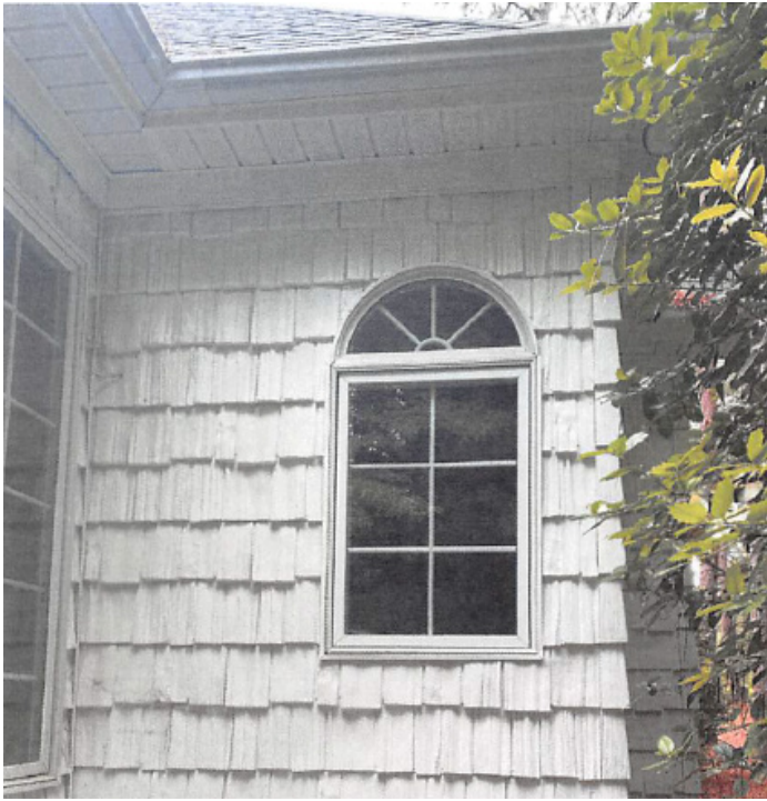
Existing Window Proposed to be Removed
