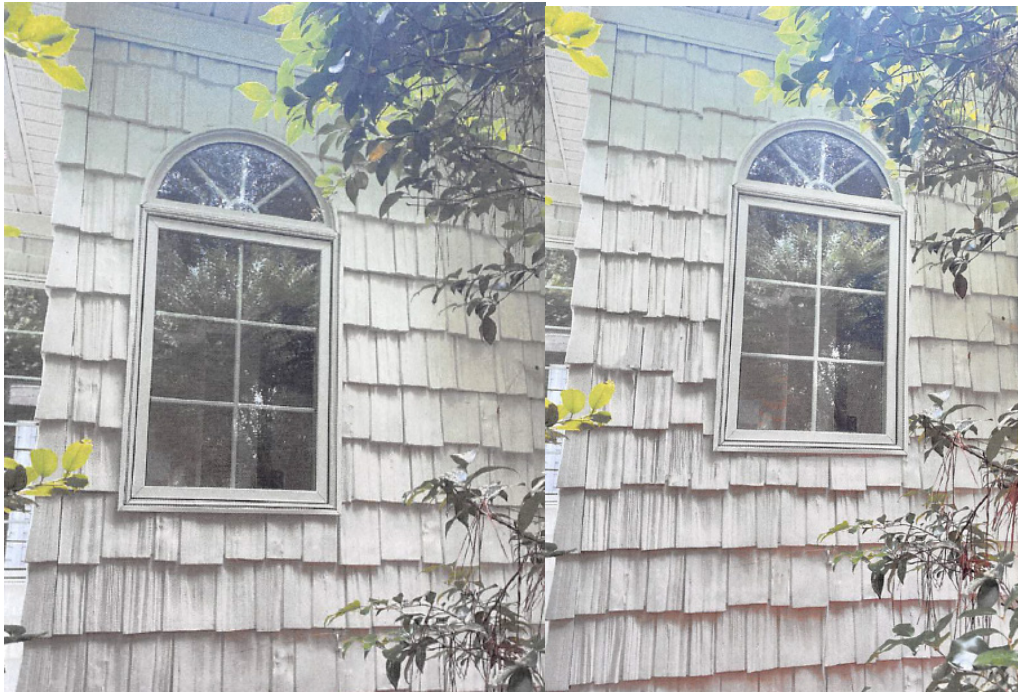
Existing Window Facing NC Hwy 5
