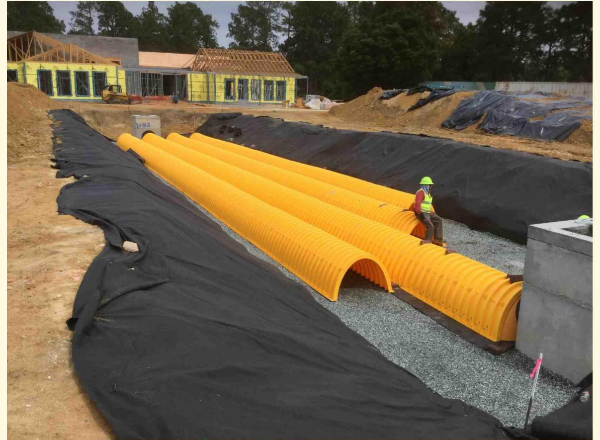
StormTech System Installation
