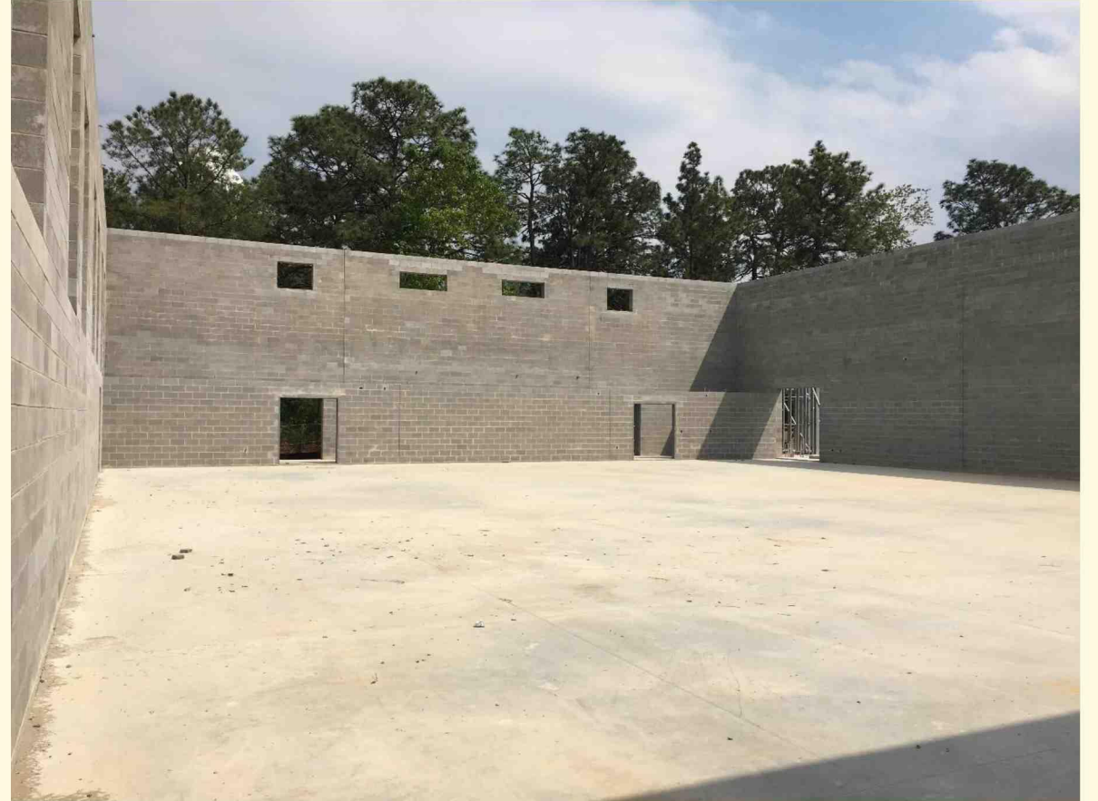
Gym in June – Ready for Trusses
