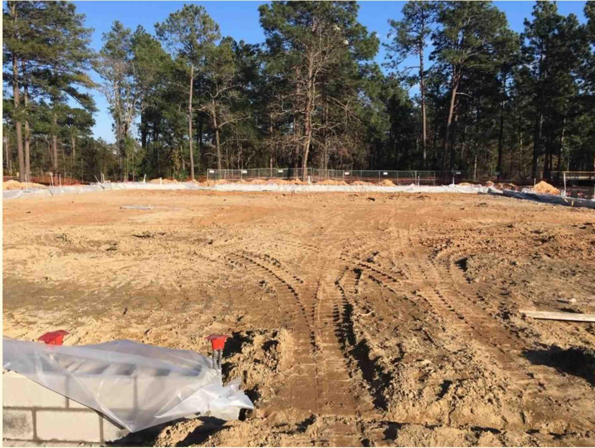
Gym Footings in March
