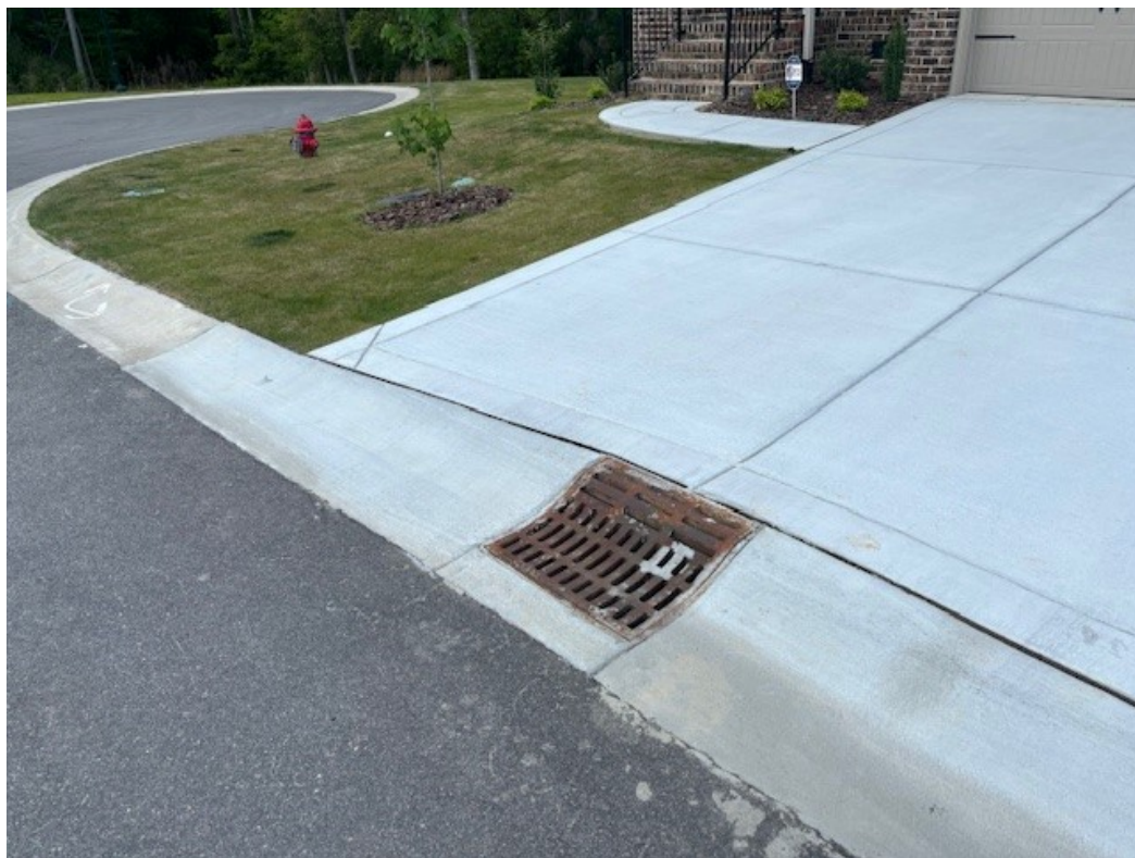
Photo 5 – Inlet Box in Valley Gutter at 156 Lark Drive
