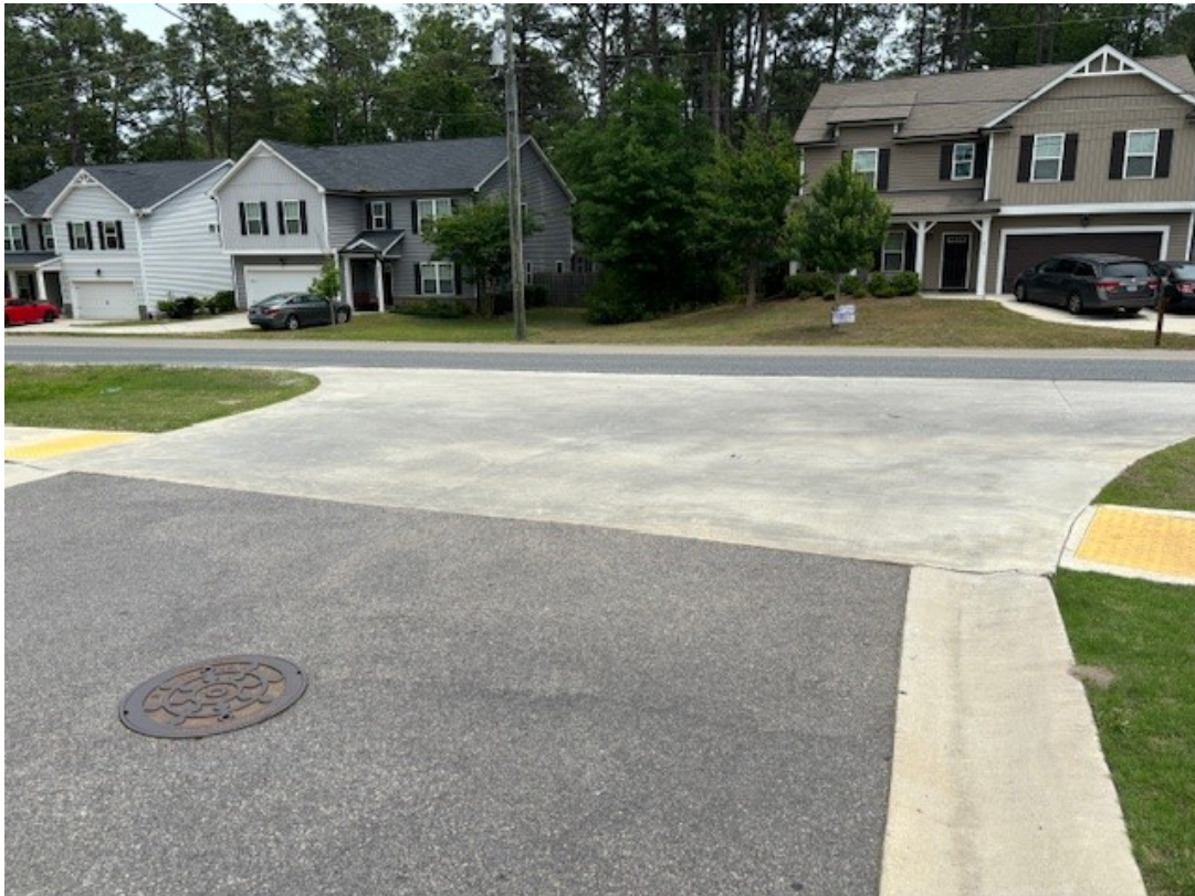
Photo 1 – Concrete Apron at Entrance off Murdocksville Road
