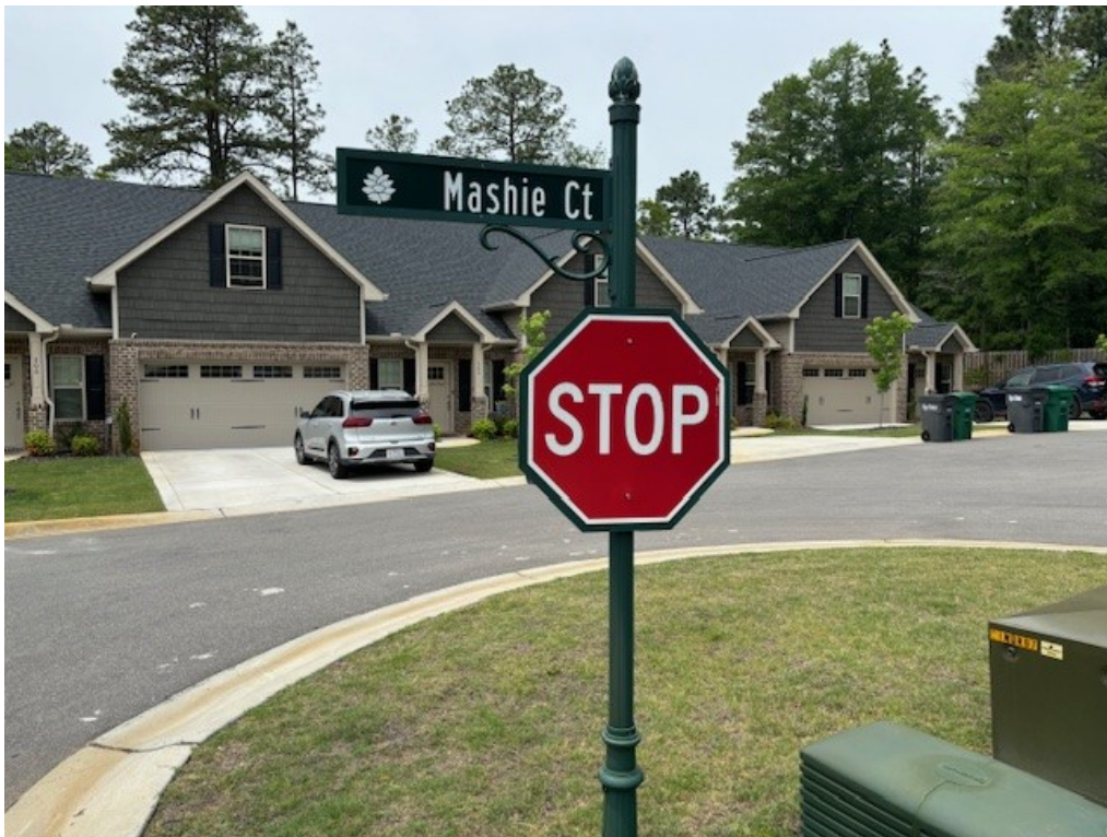
Photo 7 – Street sign and stop sign installed on same decorative post
