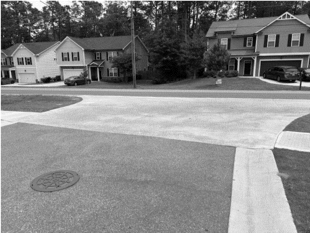
Photo 1 – Concrete Apron at Entrance off Murdocksville Road
