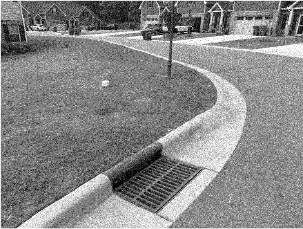
Photo 4 – Typical Curb Inlet Stormwater Box
