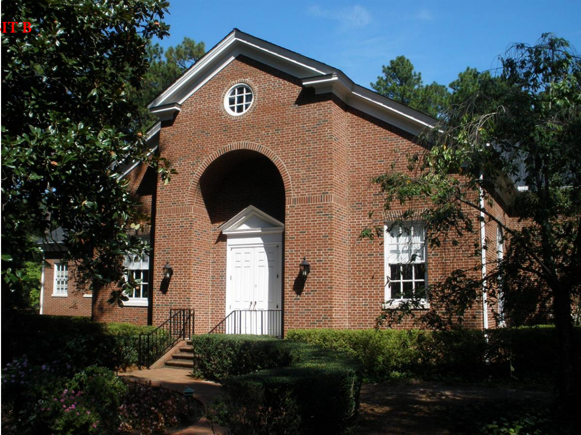
Arched Gable Entry, Chapel Hall, 1991
