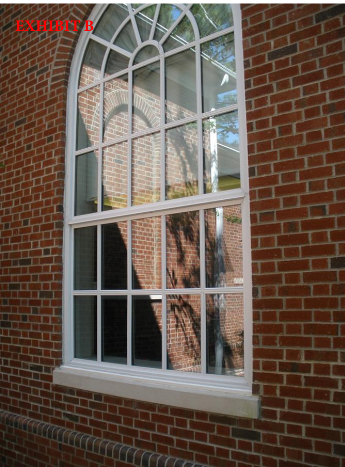
Clad Wood Windows, 1991
