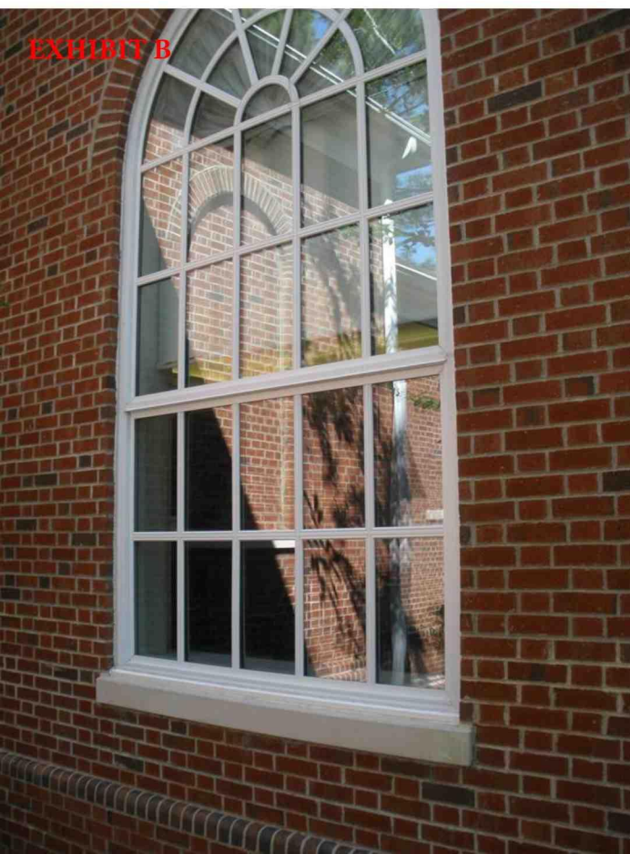
Clad Wood Windows, 1991
