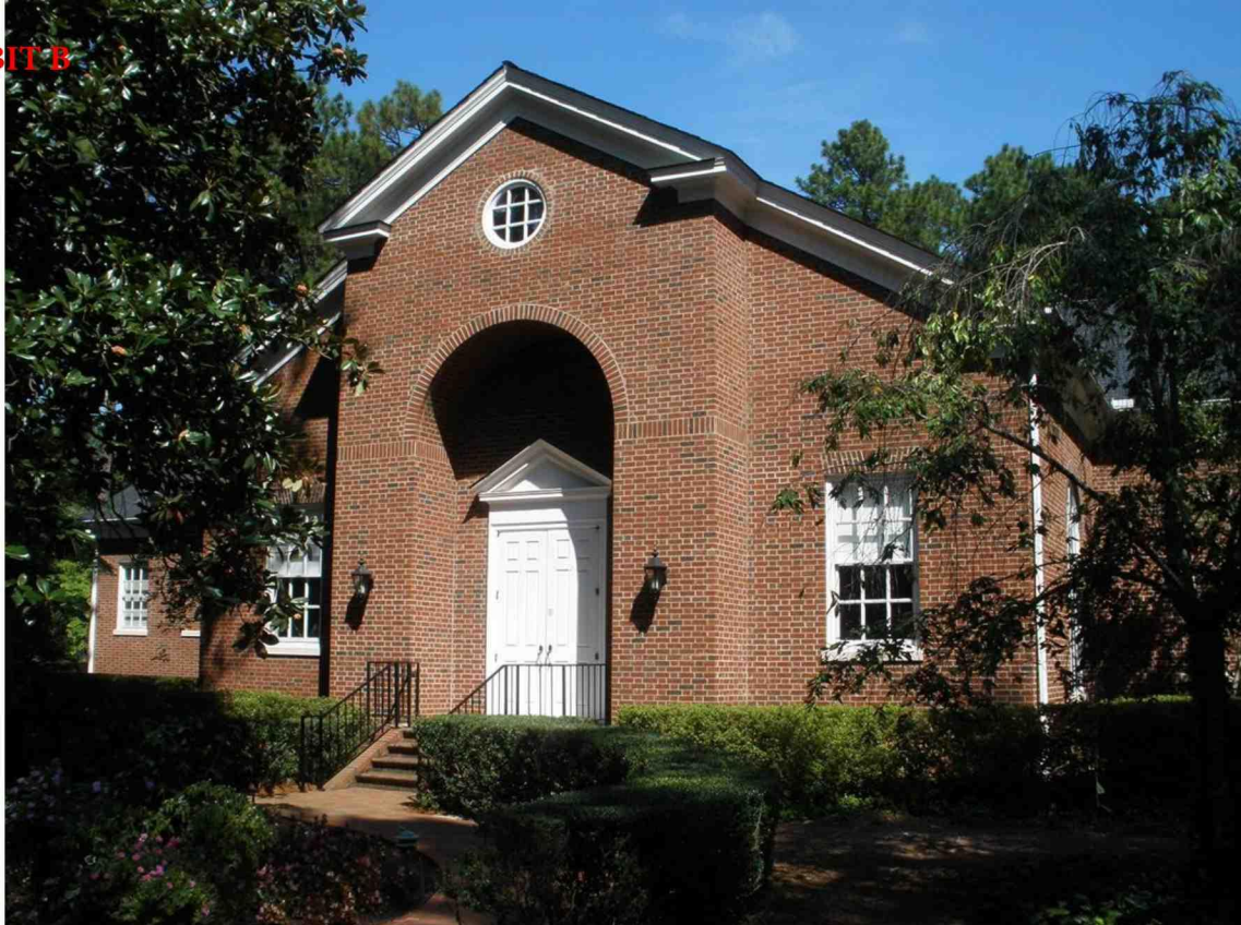
Arched Gable Entry, Chapel Hall, 1991
