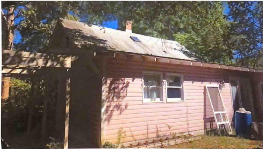
Existing Rear Roof
