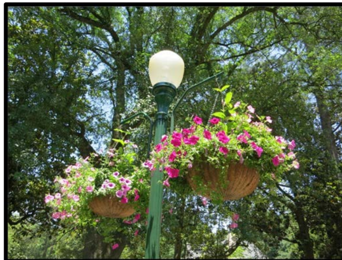
Streetlight in Village Center
