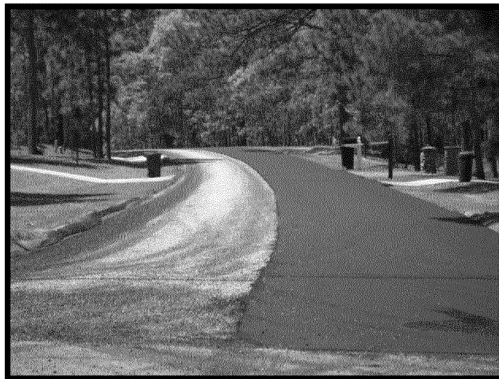
Village Street Resurfacing
