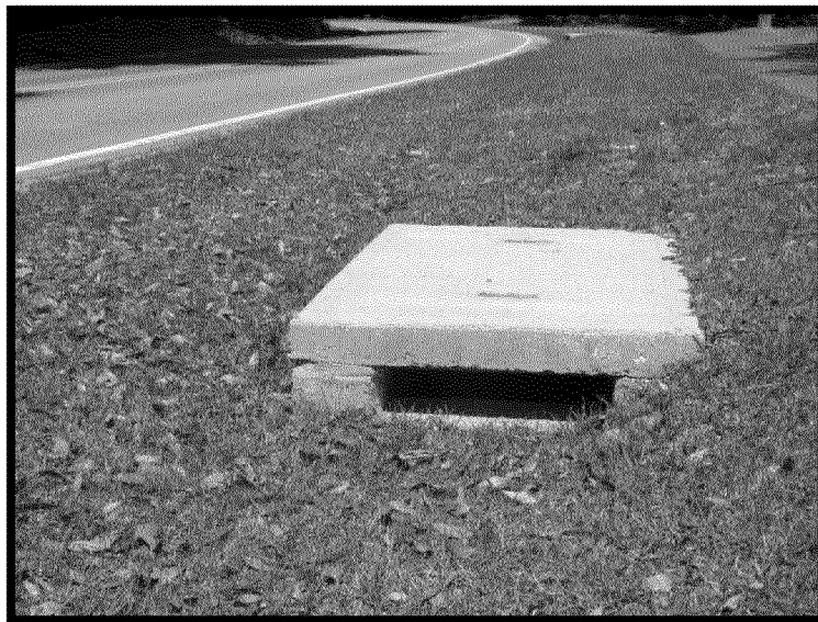
Stormwater improvement project
