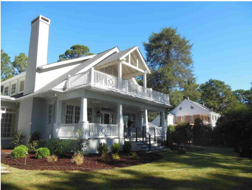
Rear porch and balcony addition
