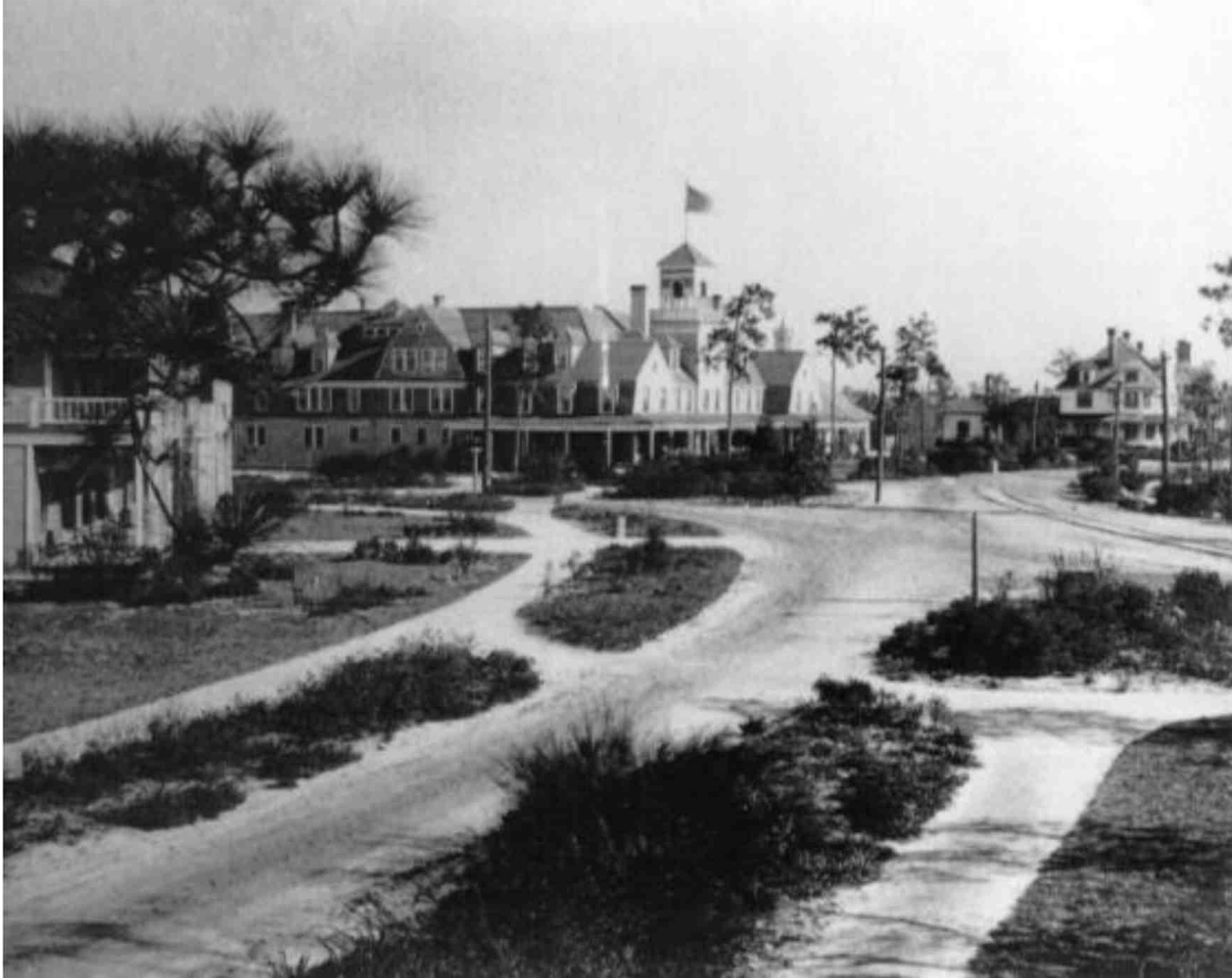
1920s Photo of clay paths and street-scaping
