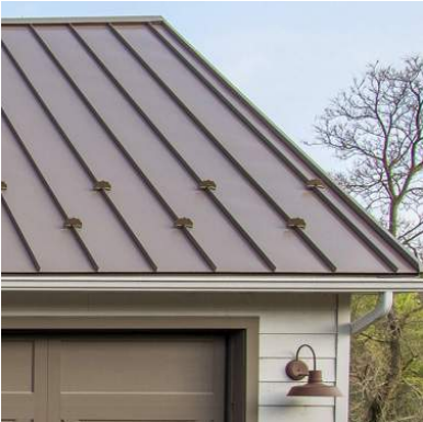
STANDING SEAM FOR FEATURE ROOF
