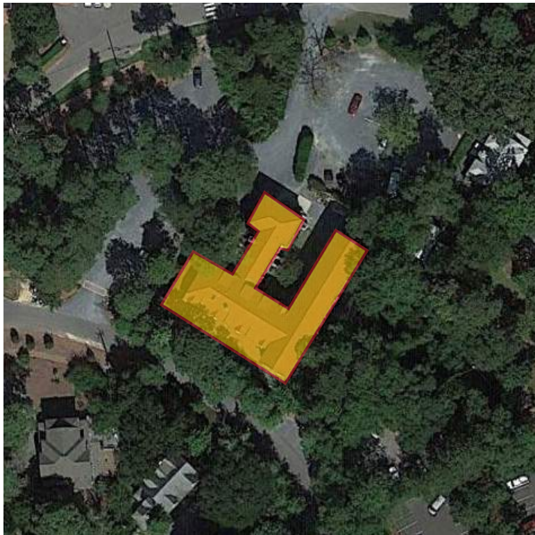
THE PINE CREST INN: 10,150 SF
