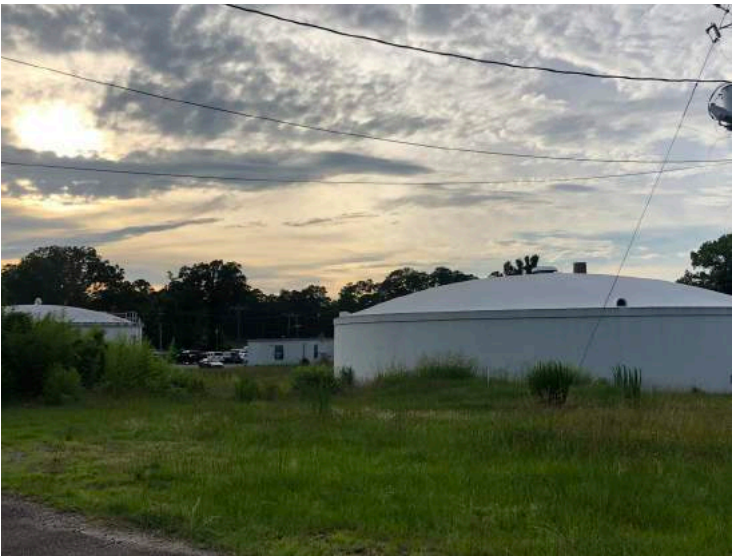
Moore County Water Tanks Source: Design Collective
