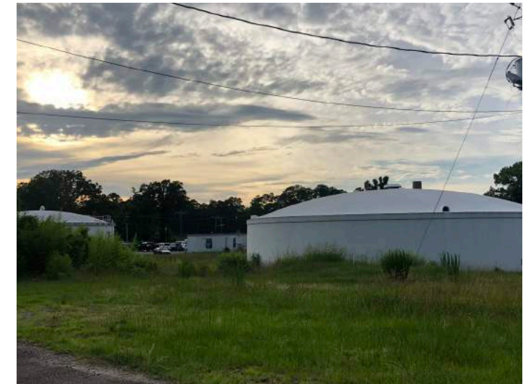
Moore County Water Tanks Source: Design Collective
