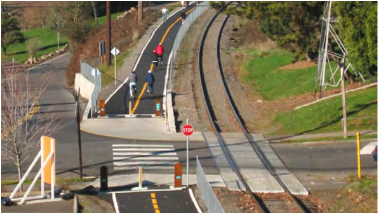
Precedent - Shared-Use Path Source: Village of Pinehurst
