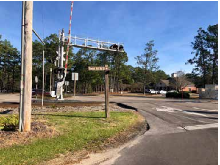
Blake Blvd Railroad Crossing Source: Design Collective
