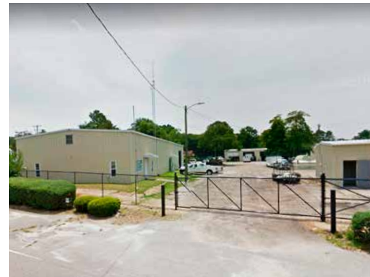
VOP Public Service Facility Source: Google
