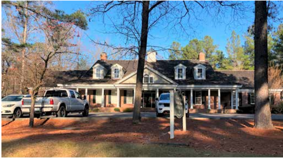
Precedent - Office - Turnberry Wood Credit: Design Collective
