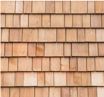
CEDAR SHAKE ROOF
