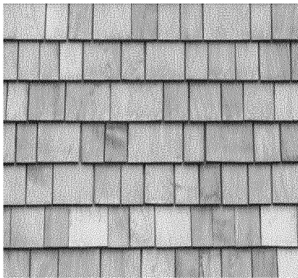
CEDAR SHAKE ROOF
