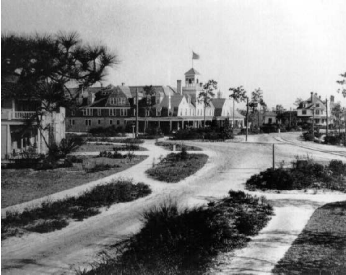
1920s Photo of clay paths and street-scaping
