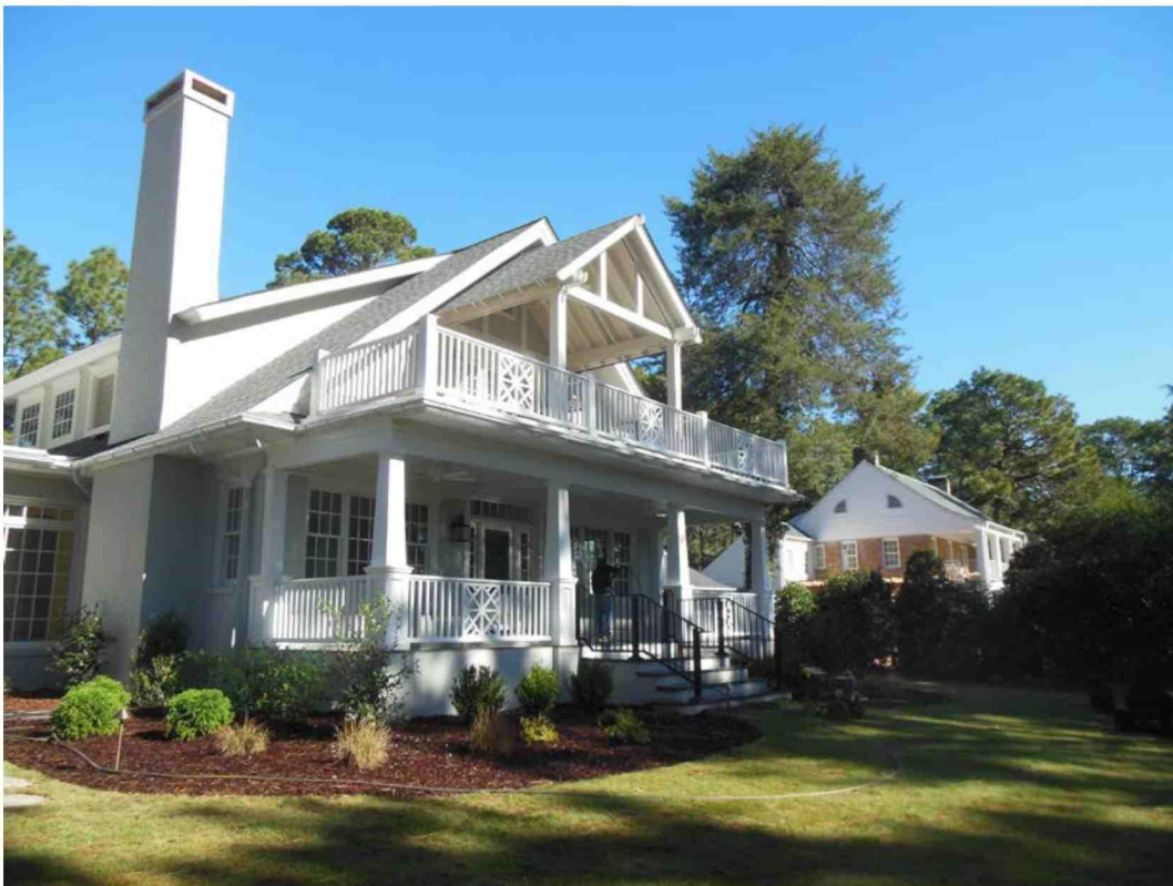
Rear porch and balcony addition
