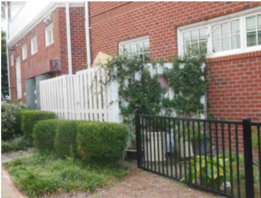
Screened commercial utility area
