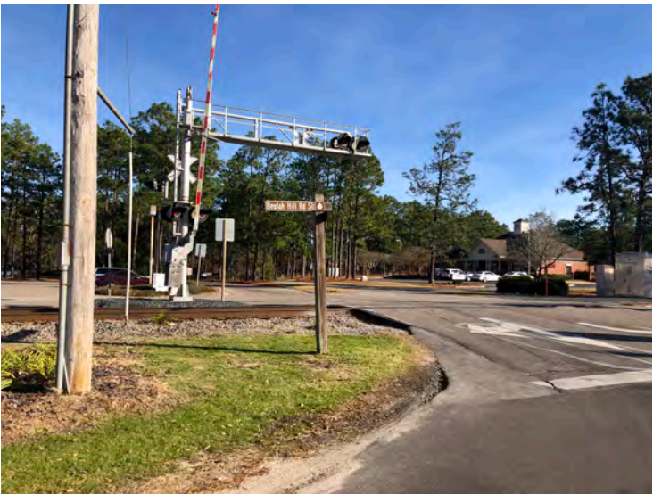
Blake Blvd Railroad Crossing Source: Design Collective
