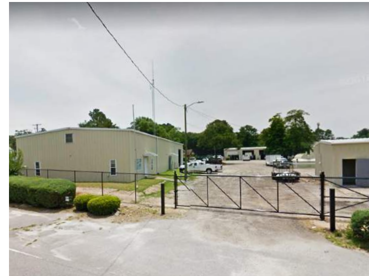
VOP Public Service Facility Source: Google
