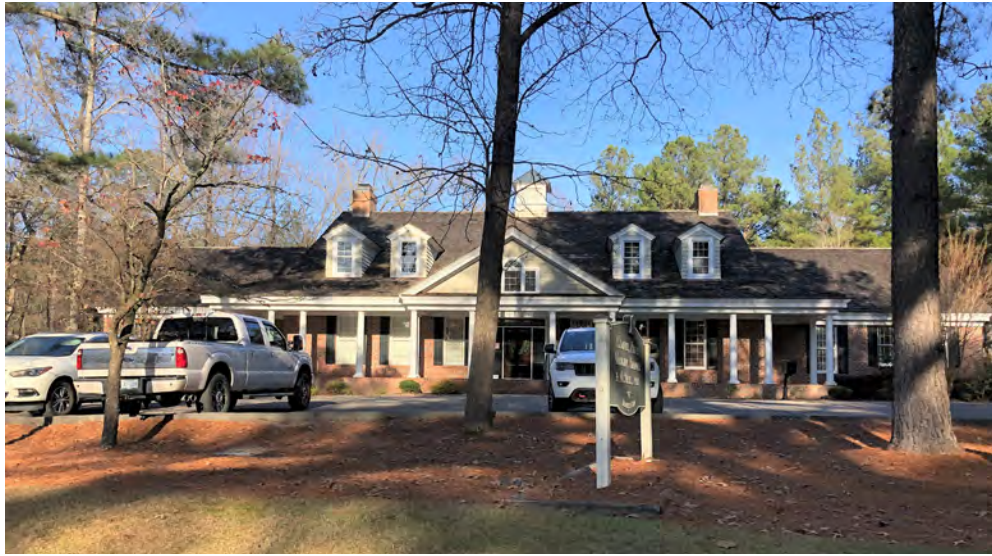
Precedent - Office - Turnberry Wood Credit: Design Collective
