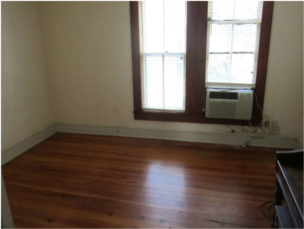
First floor apartment #1 Heart pine flooring
