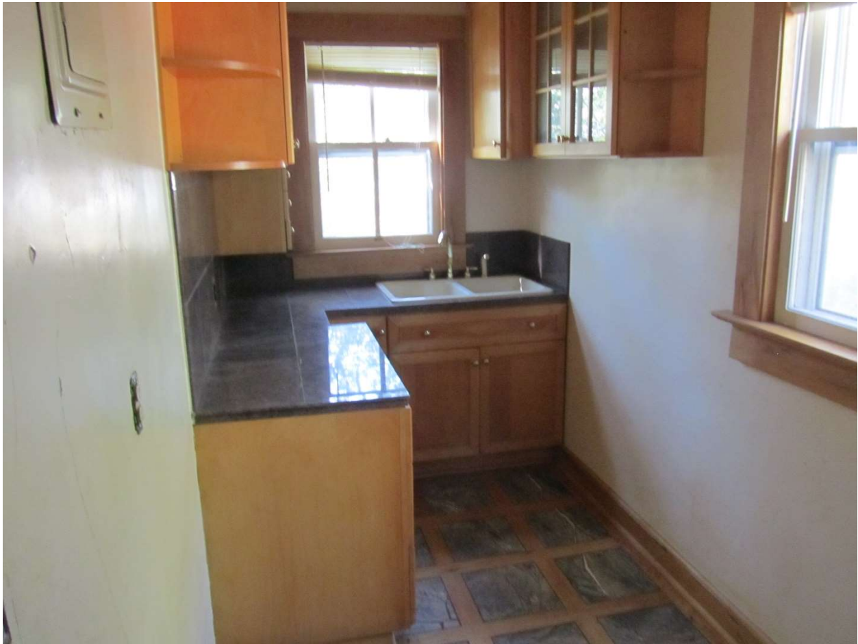
First floor apartment #1
