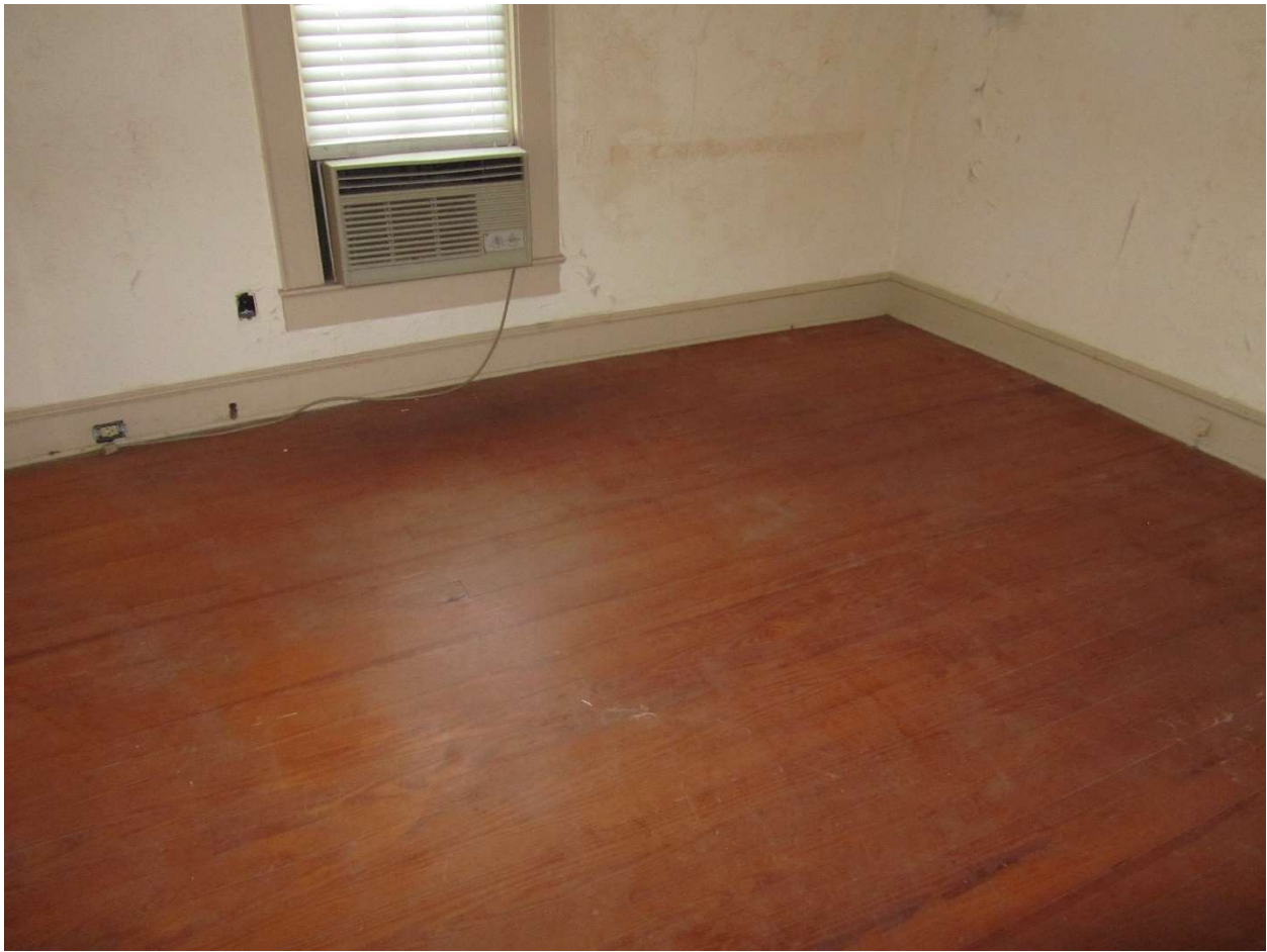
First floor apartment #2 Heart pine flooring
