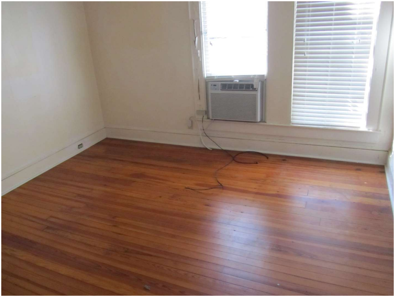
2 nd floor apartment Heart pine flooring
