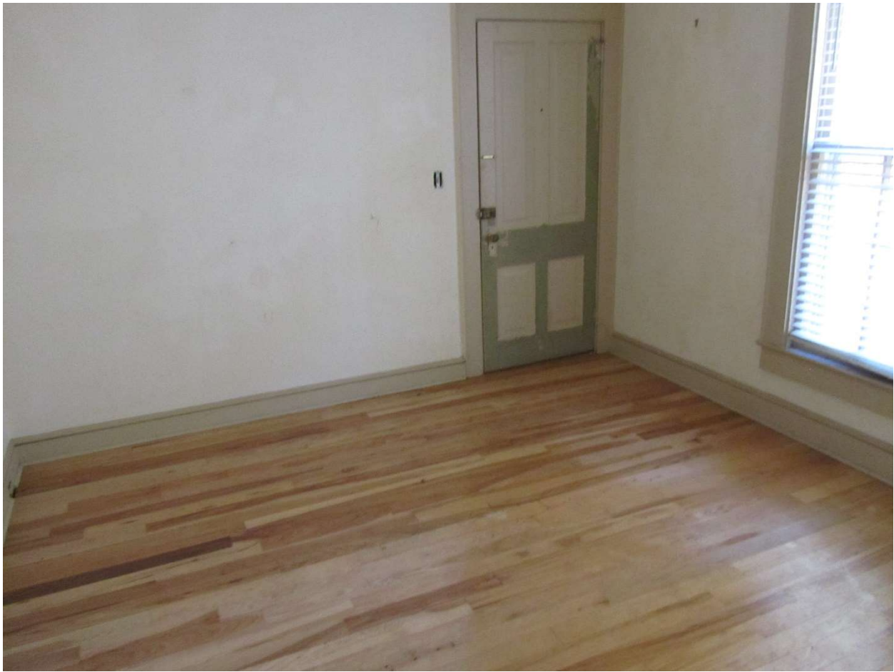
First floor apartment #2 New hickory floors
