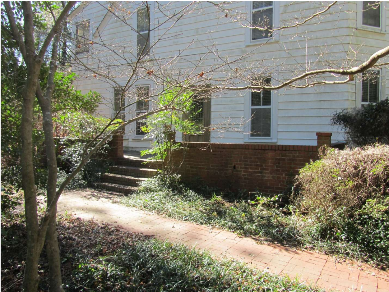
Front of house from Palmetto side
