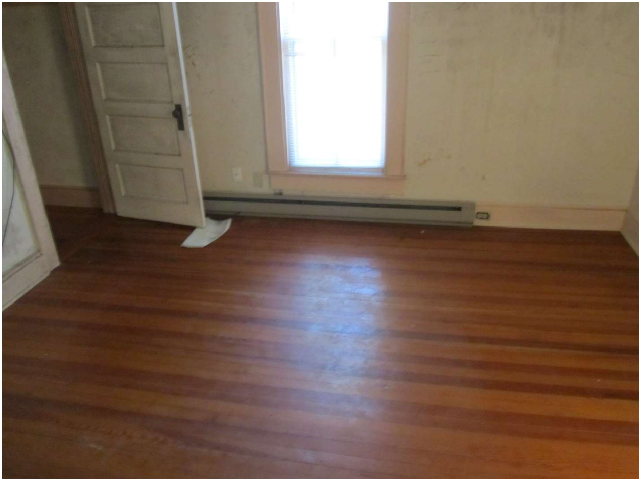
2 nd floor apartment #4 Heart pine flooring
