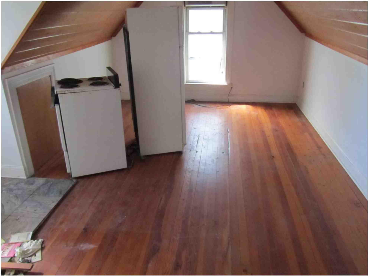
3 rd floor apartment #5 Heart pine flooring
