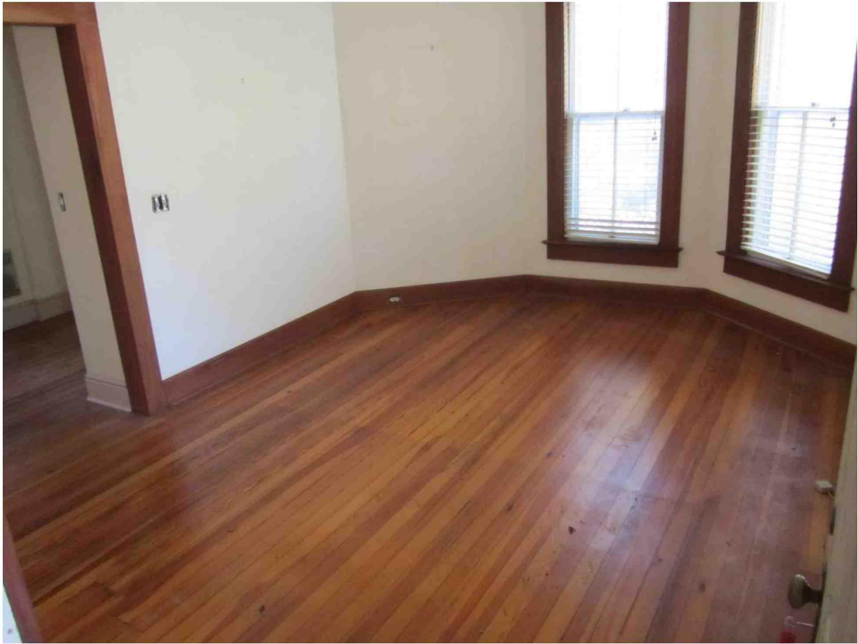
1 st floor apartment #1 Heart pine flooring
