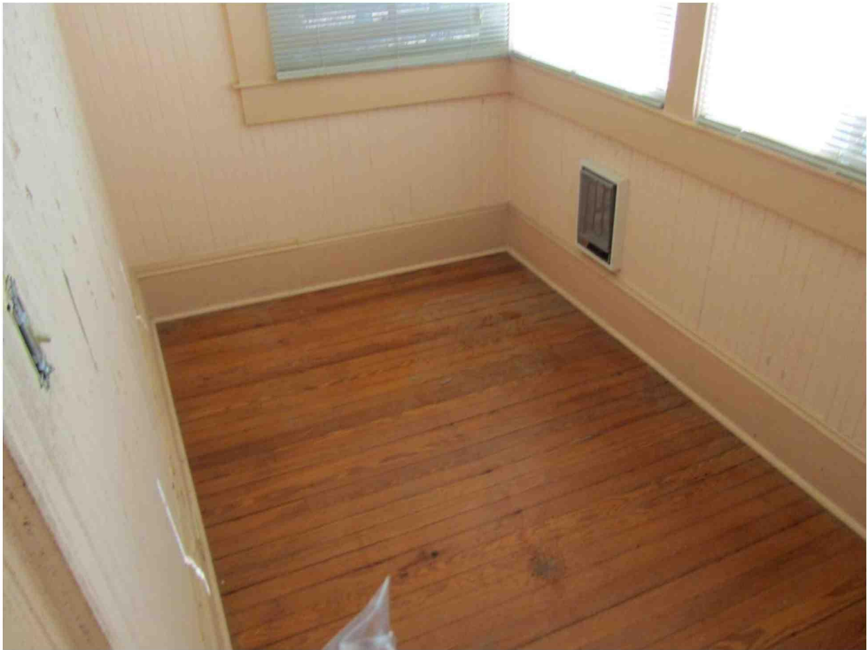
2 nd floor apartment #4
