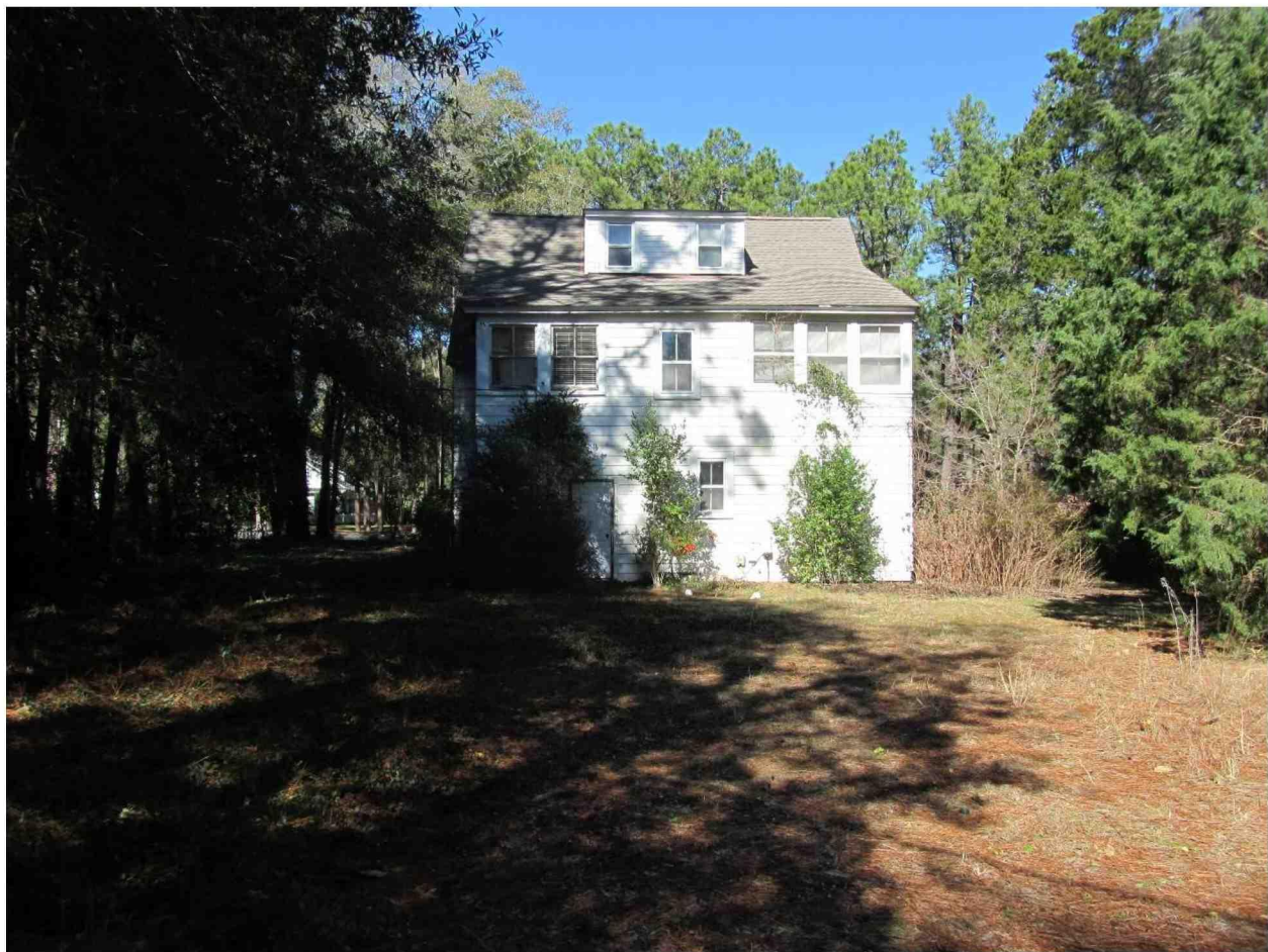
Side of house take from alley
