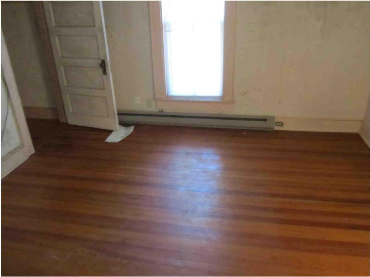
2 nd floor apartment #4 Heart pine flooring
