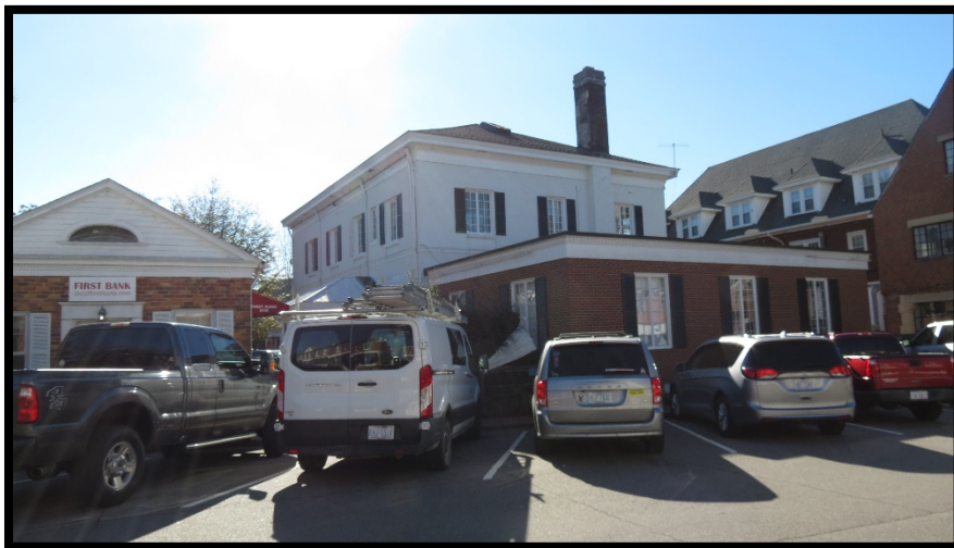
Rear Elevation Photo and Adjacent Dormer Windows
