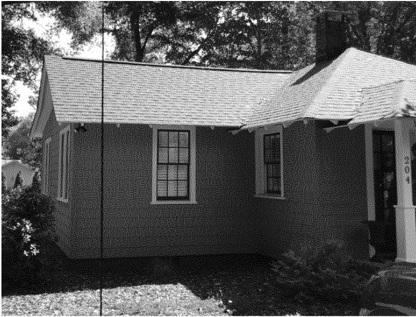
Existing Window Sash Color
