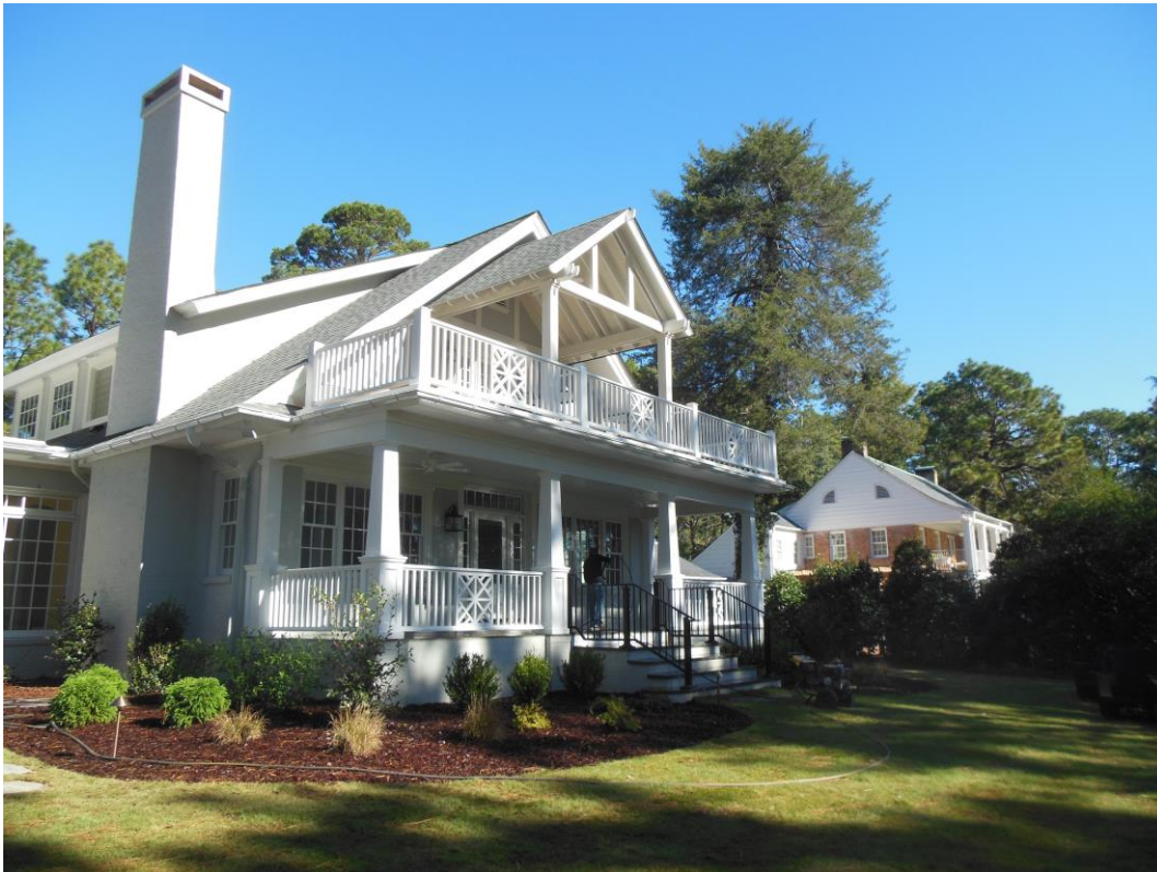
Rear porch and balcony addition
