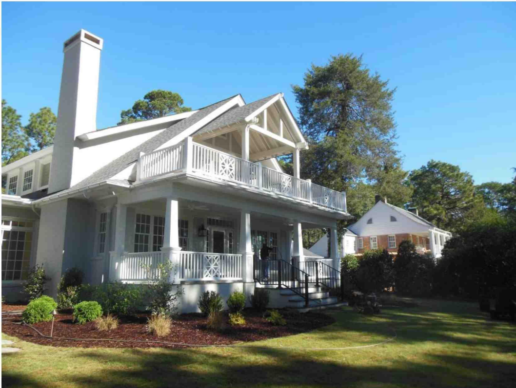
Rear porch and balcony addition
