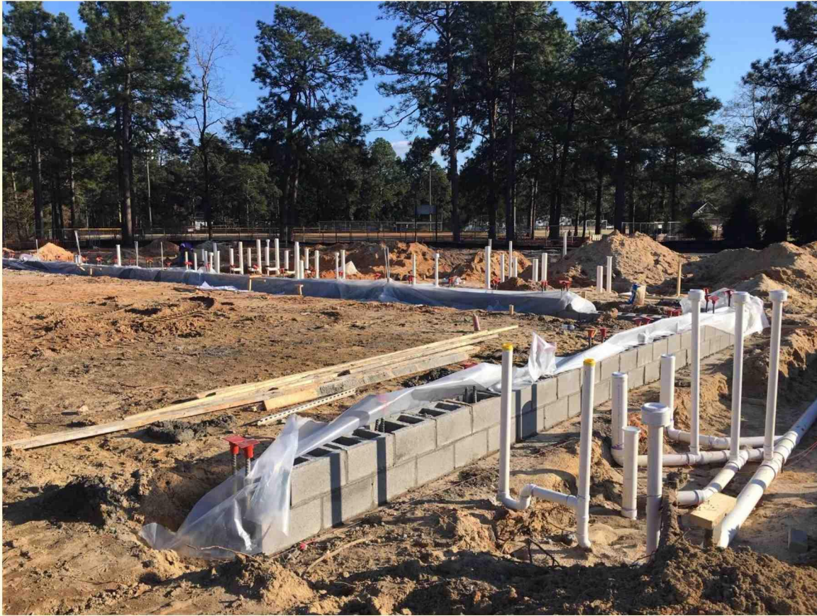
Underground Plumbing/Electrical
