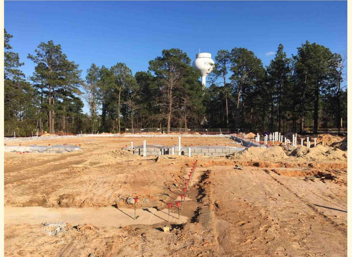
Footers & Masonry Foundation
