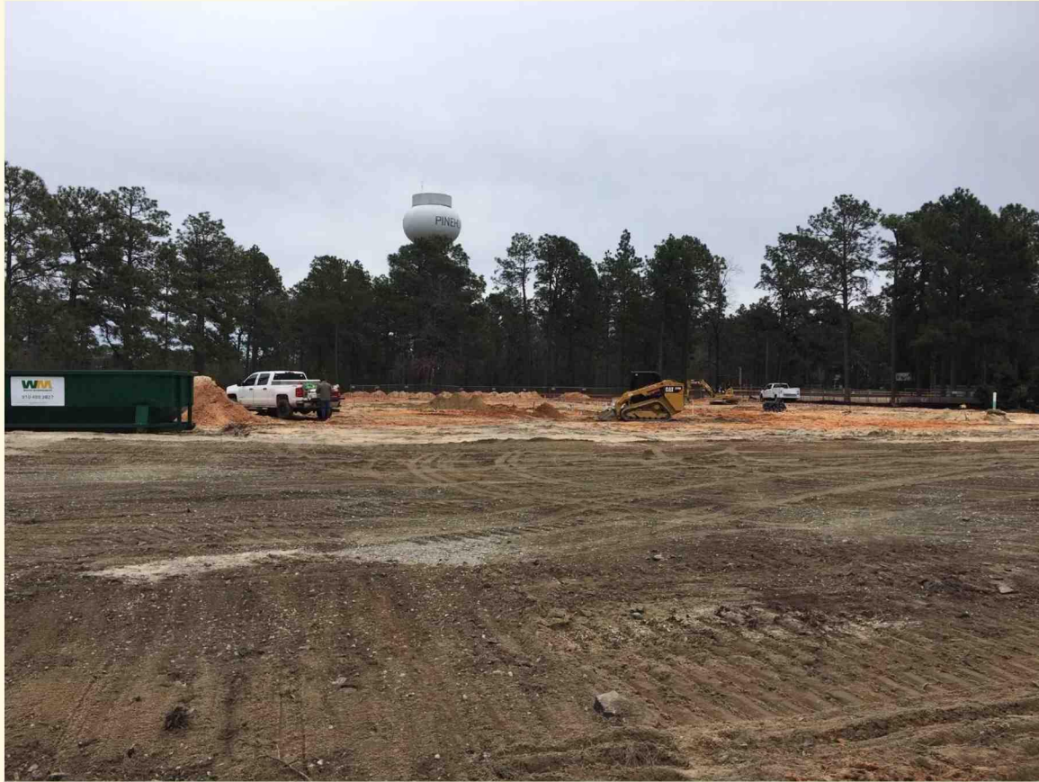
Parking Lot Grading
