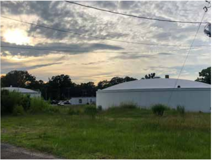
Moore County Water Tanks Source: Design Collective
