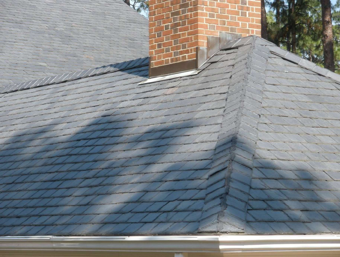
Slate Roof, 1961 shown in picture.
