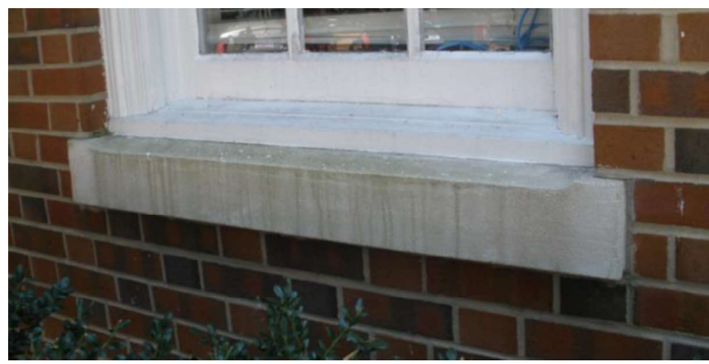
Precast Window Sills, 1961 & 1991
