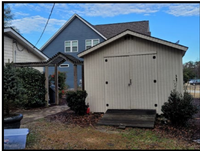
Existing Accessory Structure and Pergola
