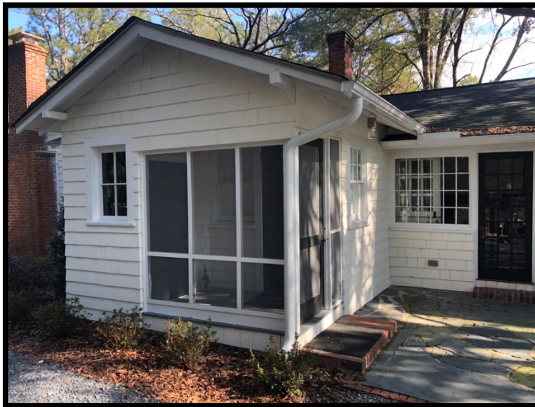
Existing Screened-in Porched to be Converted
