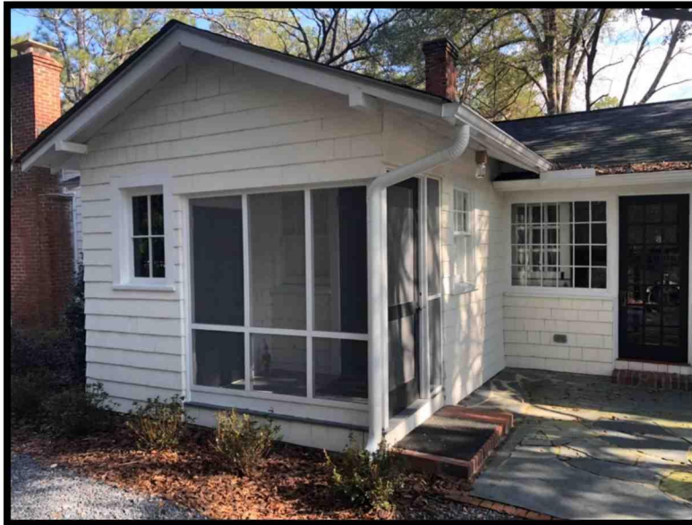
Existing Screened-in Porched to be Converted
