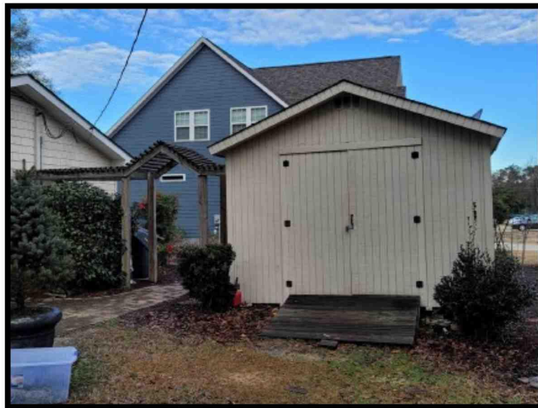
Existing Accessory Structure and Pergola
