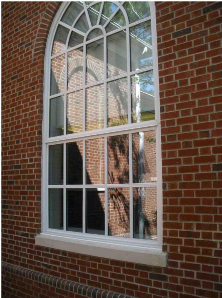
Clad Wood Windows, 1991
