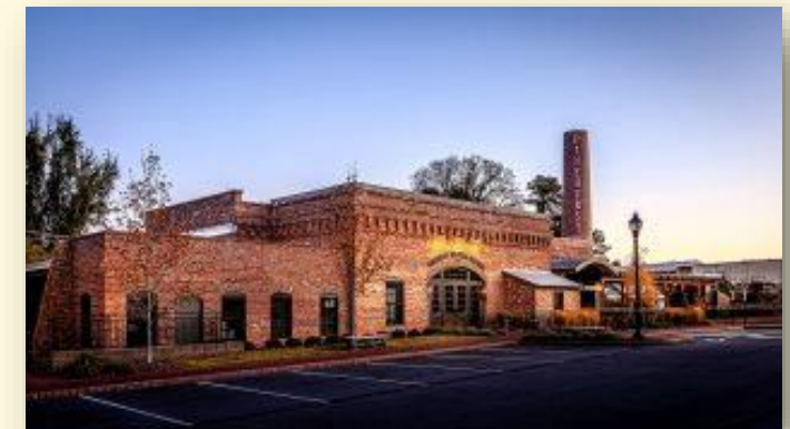
Steam Plant – After (2019)
