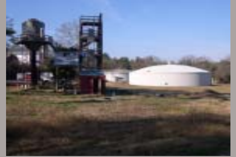
Firefighting training tower & county water tank
