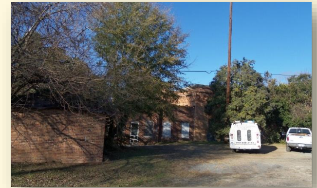
Steam Plant – Before (2013)
