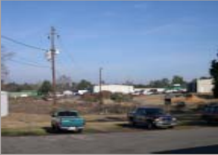
Village's public works staging area
