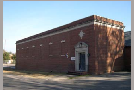
Sprint telecommunications facility
