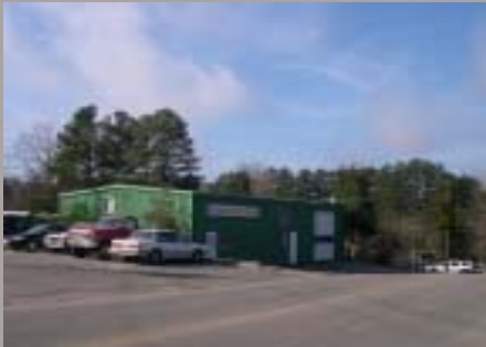
Former rescue squad facility
